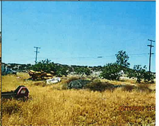
Accumulated Rubbish & Excessive Outside Stor Lpadilla
