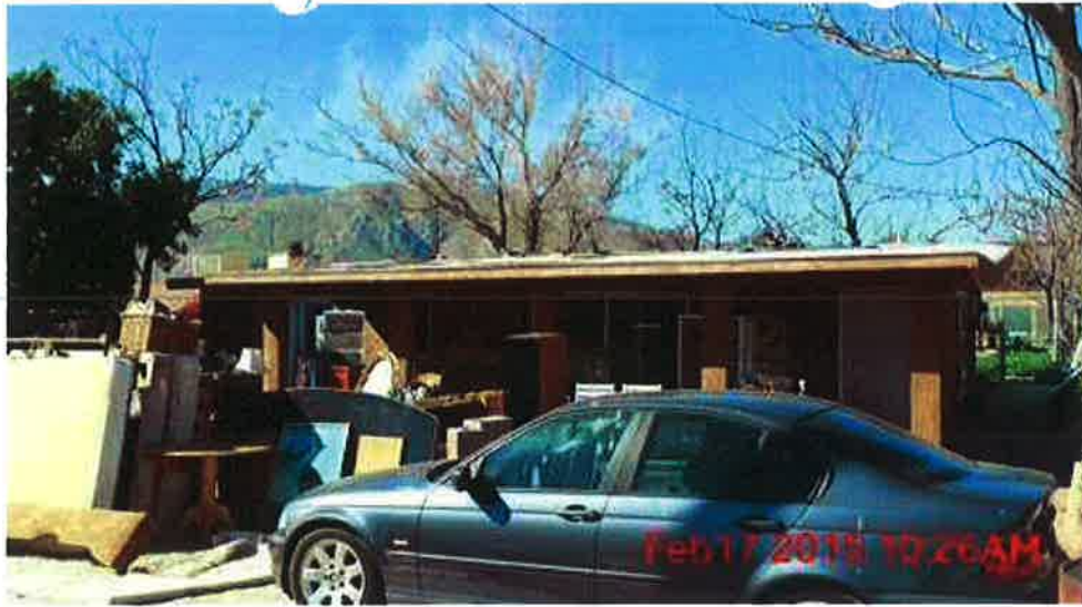
E. Torres; rubbish and excessive outside storage - 02/17/2015
