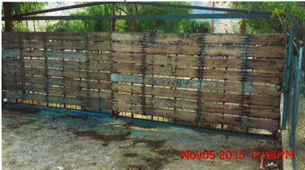
E. Torres; front gate repaired - 11/05/2015
