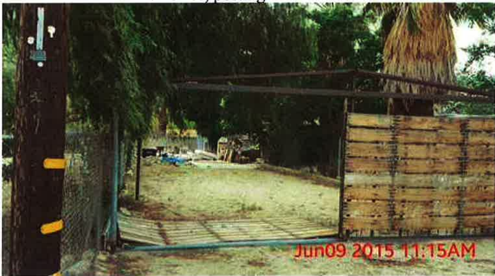
E. Torres; property remains in violation - 06/09/2015
