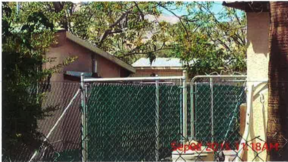
E. Torres; both substandard structures remain - 09/02/2015
