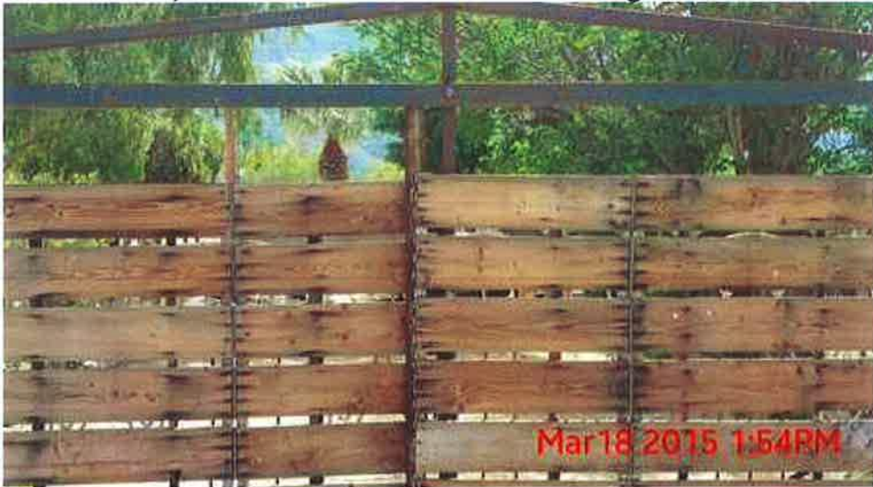
E. Torres; driveway gate - 03/18/2015
