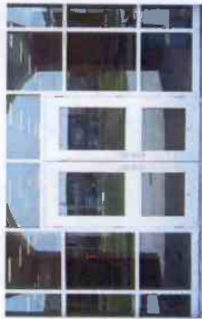
2 CLEAR ANODIZED ALUMINUM STOREFRONT ENTRY SYSTEM W/1" TEMPERED INSULATED GREY TINTED GLASS
