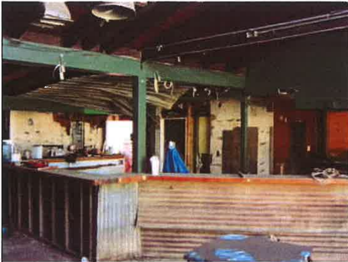
110215 TM stripped interior
