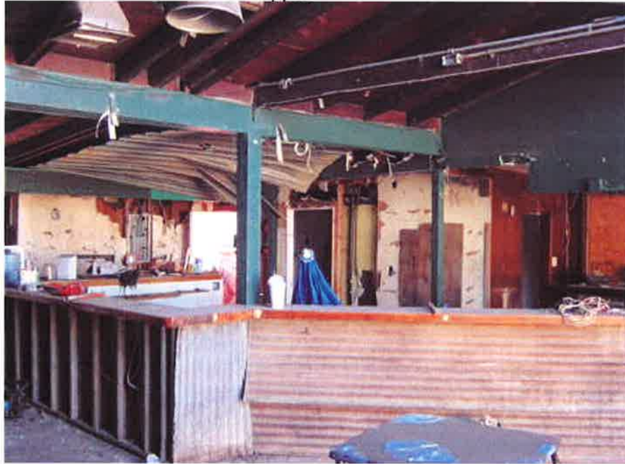
110215 TM stripped interior - 11/03/2015
