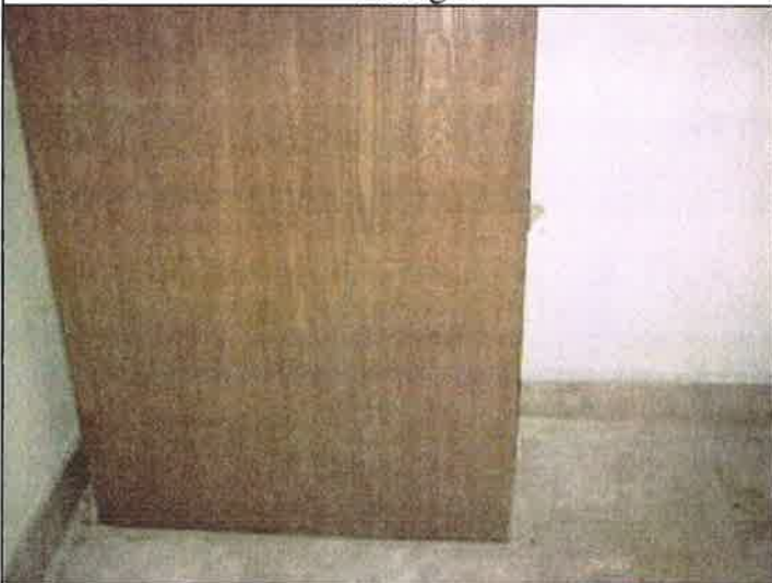
110215 TM lack of plumbing fixtures
