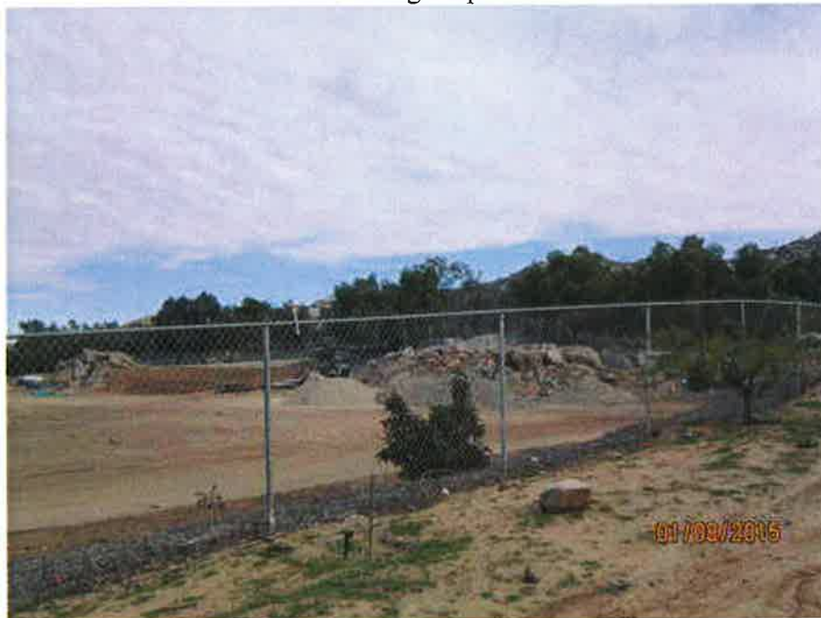
Excessive outside storage. Lpadilla - 01/08/2015
