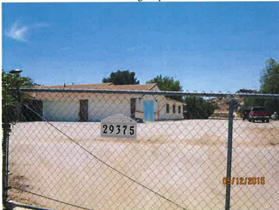
Excessive outside storage. Lpadilla - 05/12/2015
