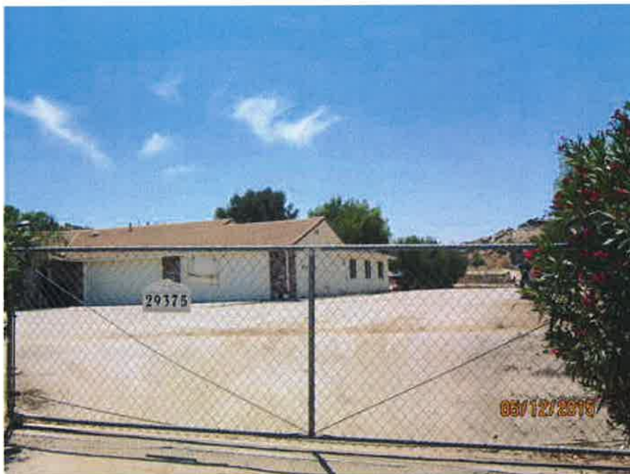
Excessive outside storage. Lpadilla - 05/12/2015
