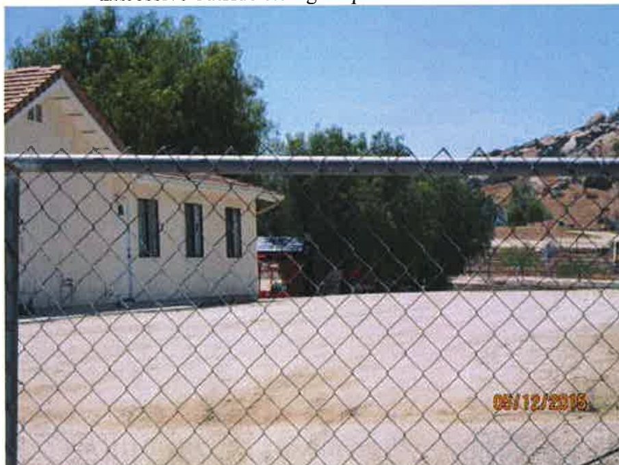
Excessive outside storage. Lpadilla - 05/12/2015
