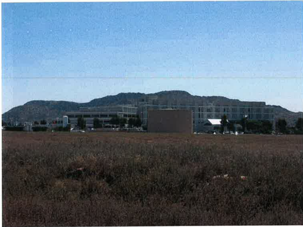
Photo 1: View of the existing Hospital facility, facing southeast from the northern border of the project site.
