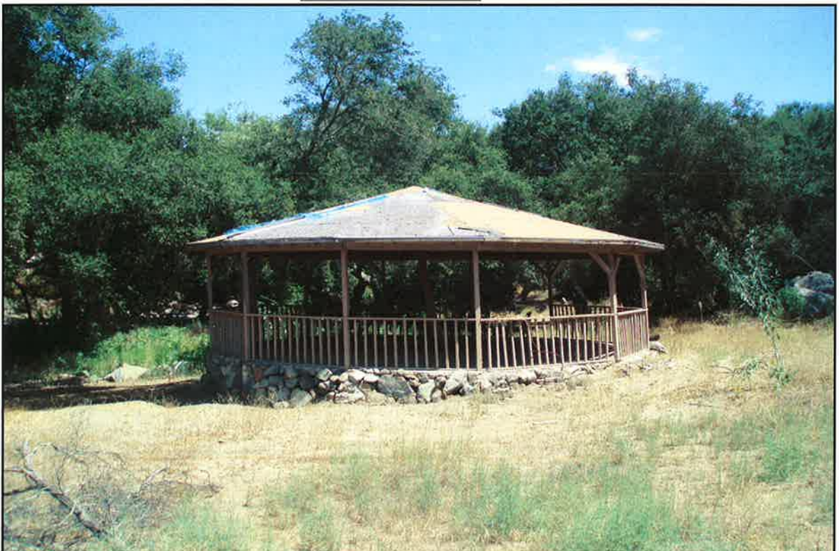
PHOTO # 10 DATE: 7/23/09 TIME: 1300 PM TAKEN BY: BF #21
