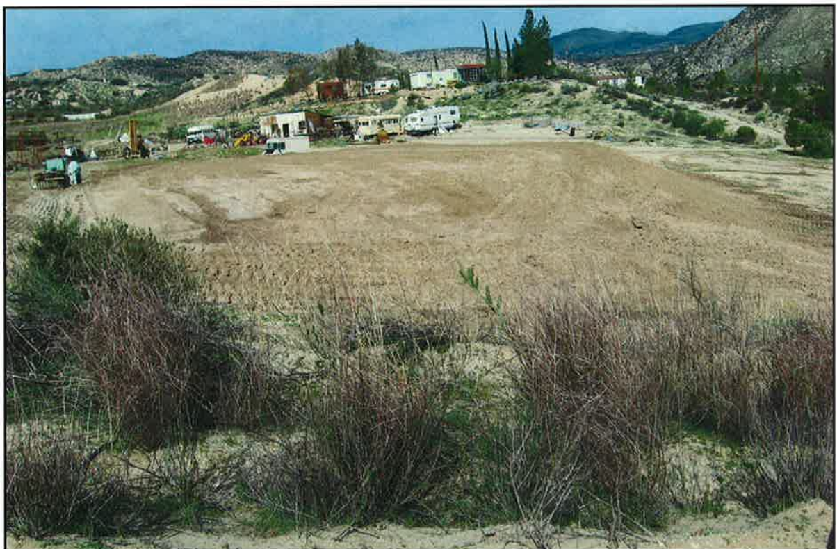
PHOTO #6 Clear view of pad.
