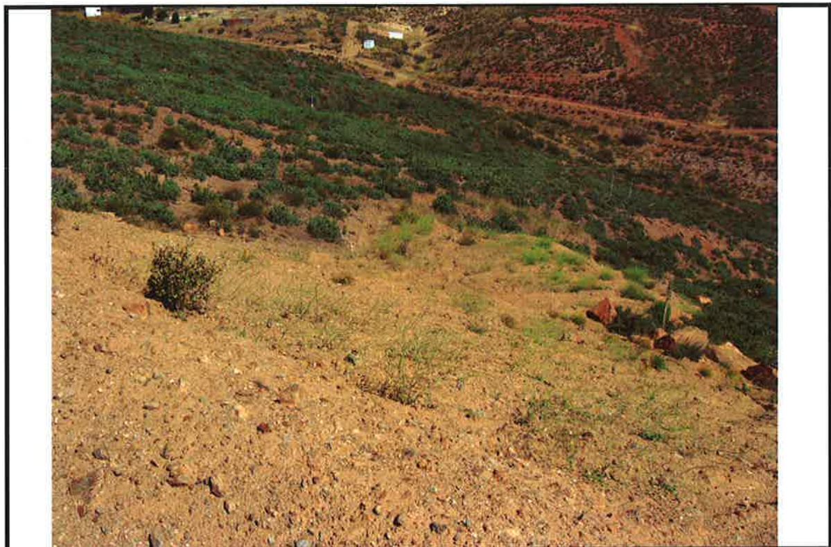
PHOTO # 4 DATE: 07/07/09 TAKEN BY: J. Pike #59 NOTES: Violation has slid onto another lot.
