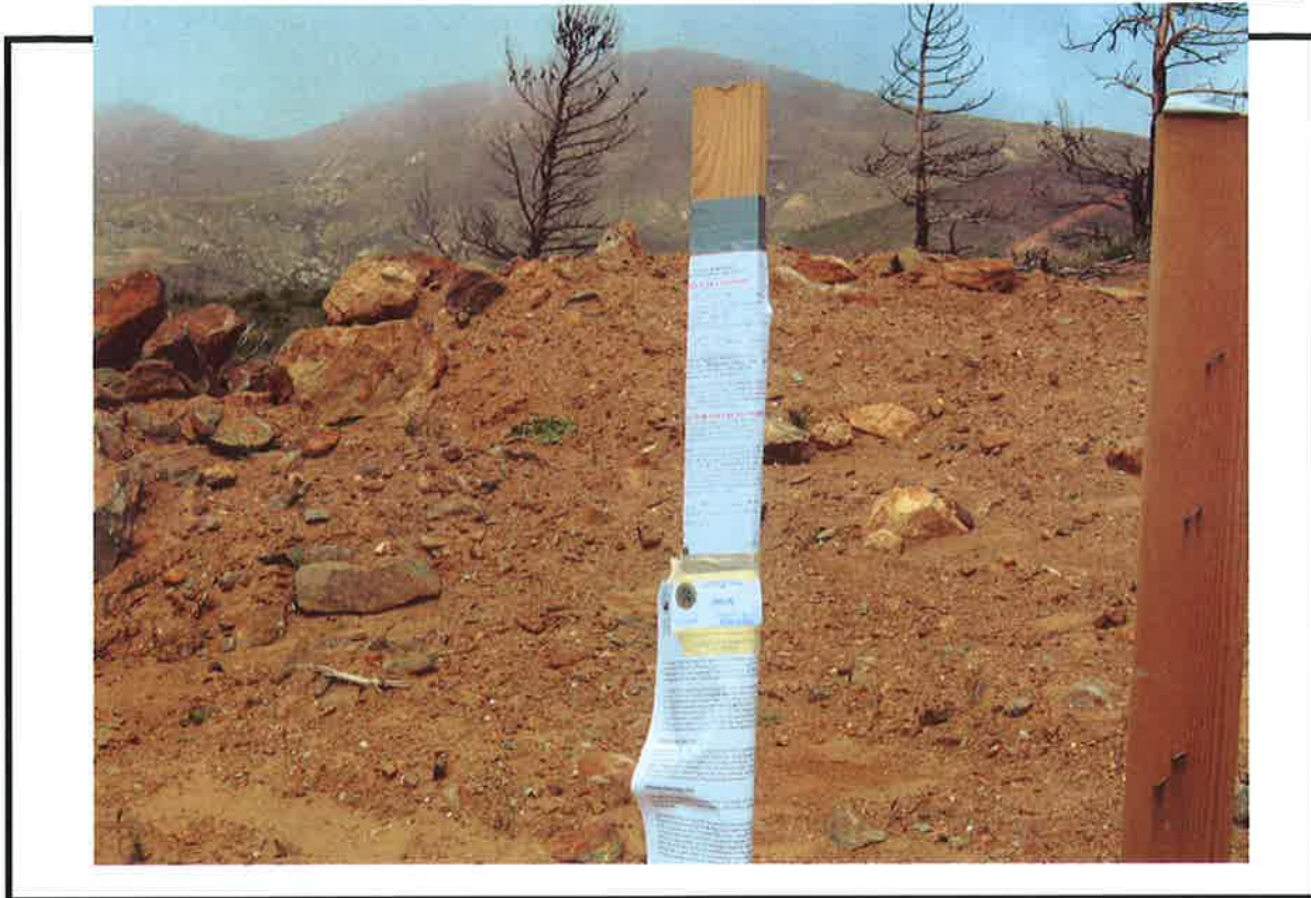
PHOTO # 11 DATE: 05/07/08 TAKEN BY: A Green#69 NOTES: posting of grading violations and grading flyer, and business card.
