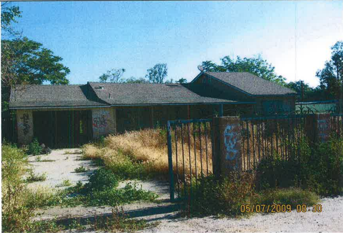
CV079901 14545 CHANDLER STREET SSS, EOS AND AR - RE-INSPECT AND POST NOTICES FRONT DRIVEWAY GATE OPENED AND ACCESSIBLE ALL {00} PHOTOGRAPHS TAKEN ON MAY 7, 2009, BY DONNA PAYNE #58
