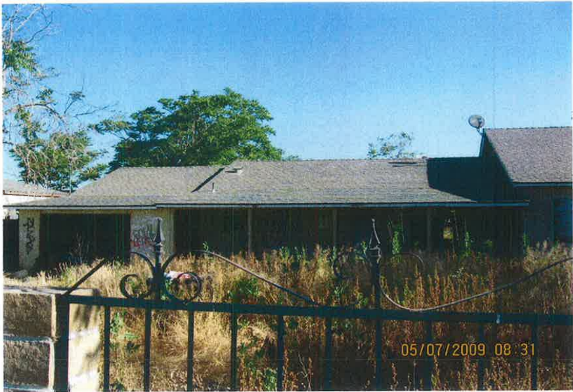
THIS PHOTOGRAPH SHOW THE PROPERTY IS COVERED WITH GRAFFITI
