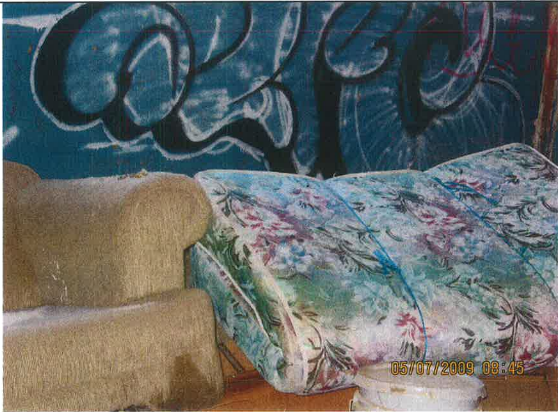
THIS IS THE FIRST ROOM IN THE UNPERMITTED ROOM ADDITION NEAR THE GARAGE
