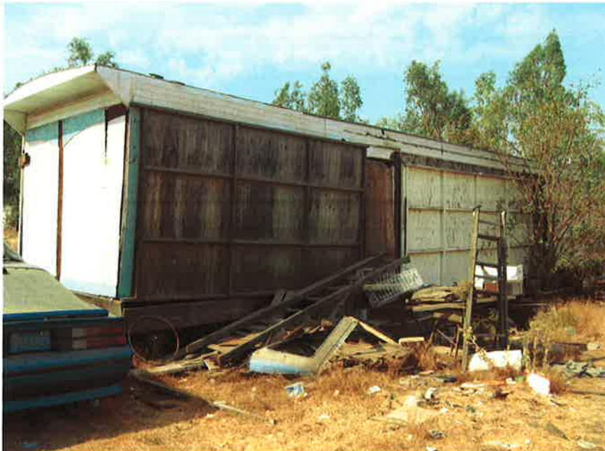
Photo #26 – trash and debris
