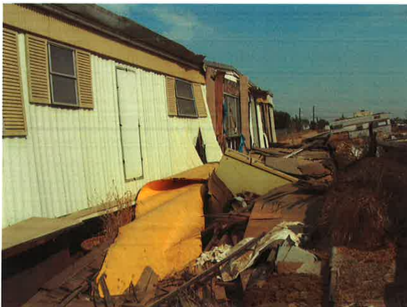
Photo #30 – more demolition debris and trash
