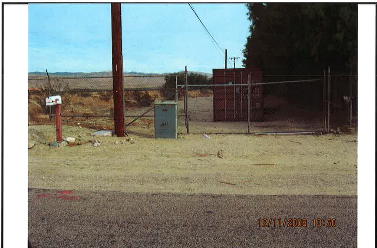
PHOTO # 8 TAKEN BY: D Jurden, CET ADDRESS: 1 par S/O 18850 Paintbrush Trail NOTES: Photo taken from right of way on Bubbling Wells Road
