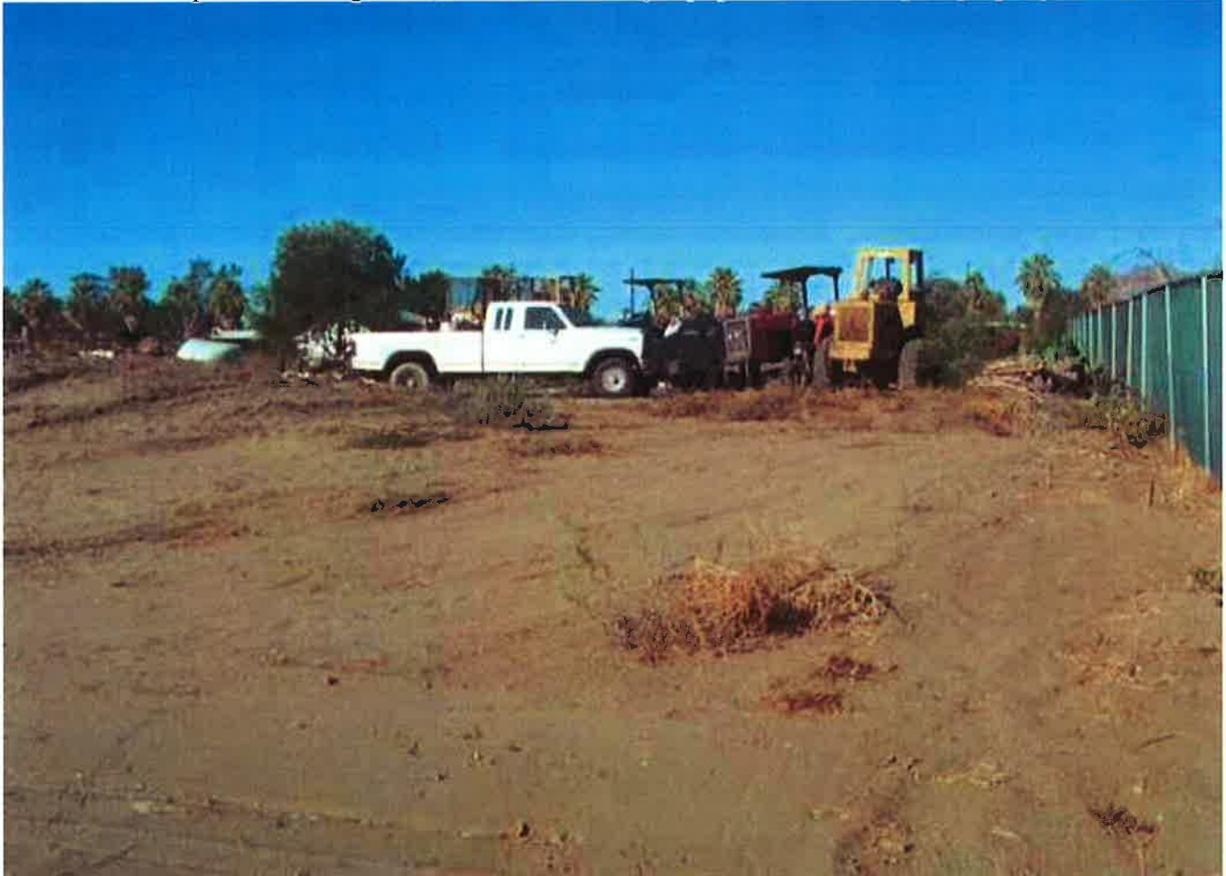
Overview of photo #5 prior to zooming in. North side of the property. - 10/05/2009
