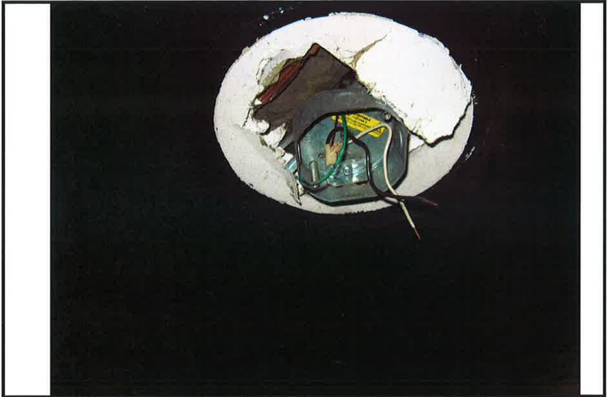
PHOTO # 7 DATE: 01/08/08 TAKEN BY: A Green#69 NOTES: exposed electrical wires N.O.D. #6
