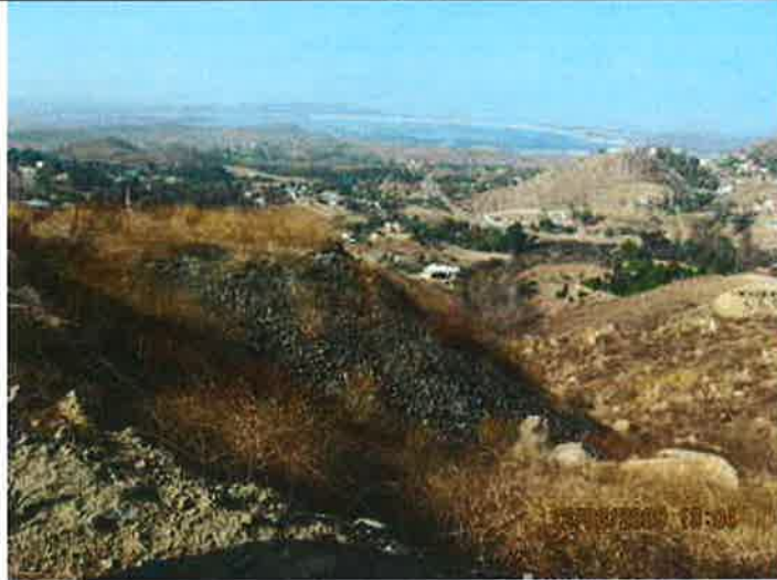
Grading on hillside
