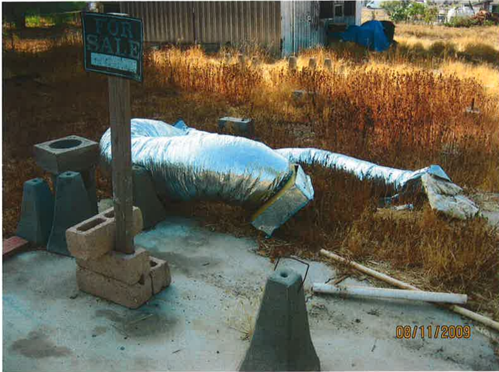
PHOTO # 3 NOTES: AR – Area # 3 - used ducting measured 6' X 6'
