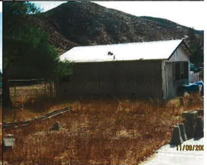
R Ryder - Substandard Structure remains on the property
