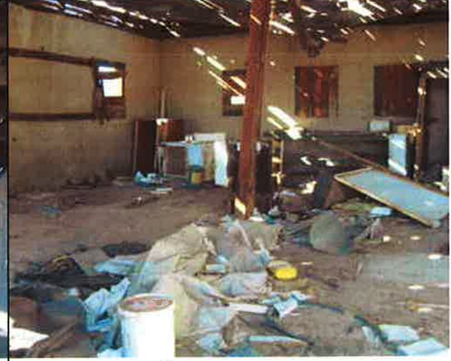
Structure # 1 - Garage Defect # 10, 11, 13, 14 &
