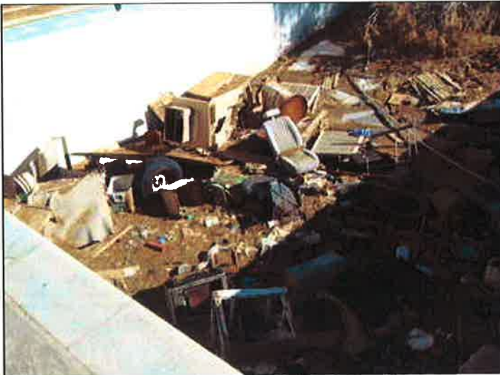
Accumulated Rubbish In Pool
