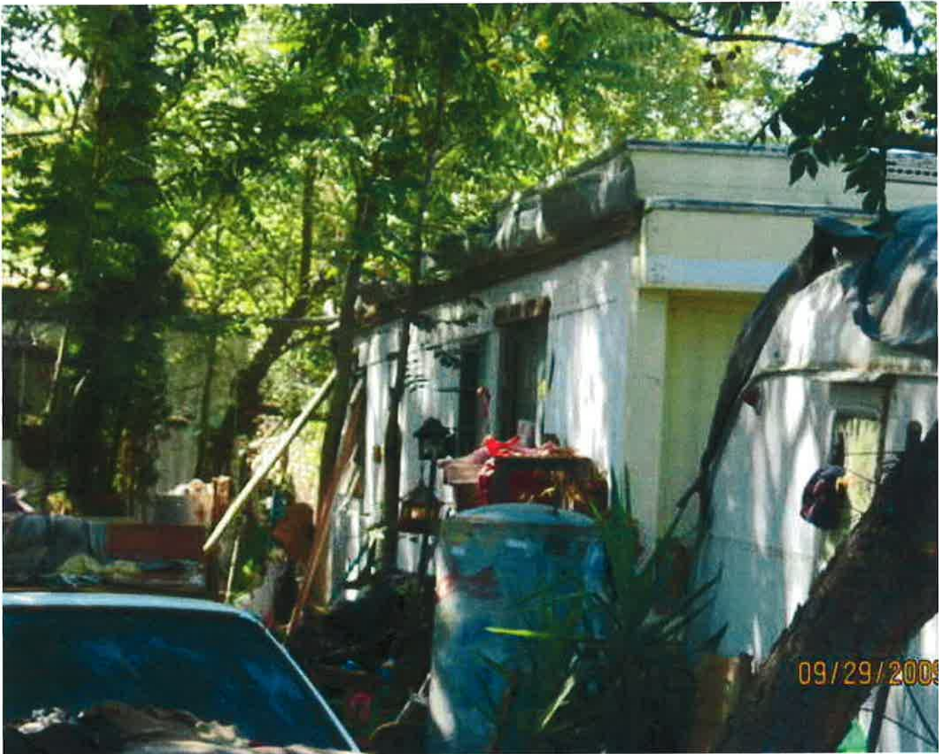
R Ryder violations remains - 09/30/2009
