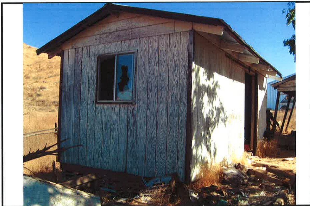
PHOTO # 13 DATE: 10/15/2008 TAKEN BY: LPADILLA 26580 PEACH ST, STRUCTURE # 3 SHED
