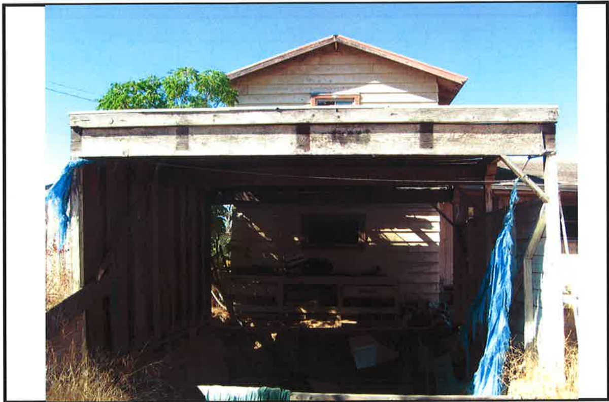
PHOTO # 11 DATE: 10/15/2008 TAKEN BY: LPADILLA 26580 PEACH ST, STRUCTURE 2 CARPORT AT DWELLING
