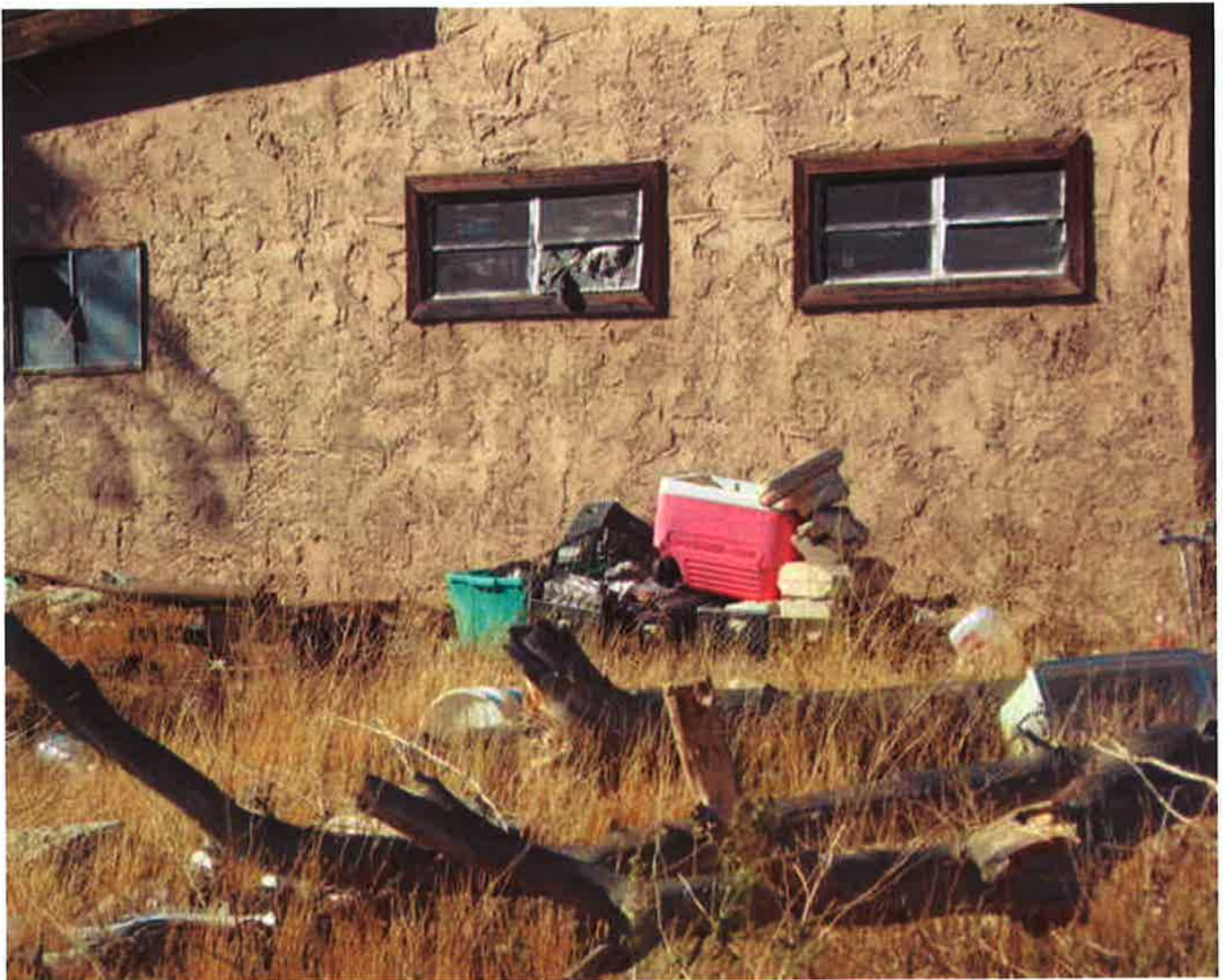
IMG_7035.JPG - 11/16/09 Rubbidh remains on property. - 11/18/2009
