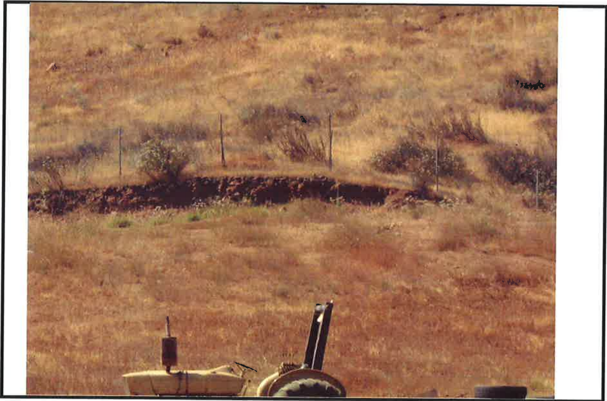
PHOTO # 3 DATE: 7/21/09 TIME: 10:05 HRS TAKEN BY: J.Morris Grading without Permit
