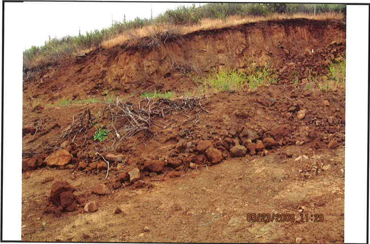
PHOTO # 1 TAKEN BY: D Jurden, CET ADDRESS: 20775 Gardenias Street NOTES: Photo showing recent grading
