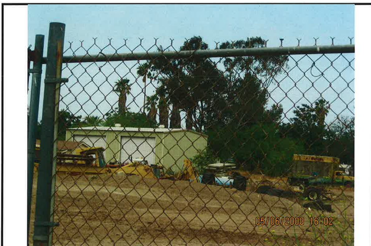
PHOTO #1 Notes: Construction equipment on property
