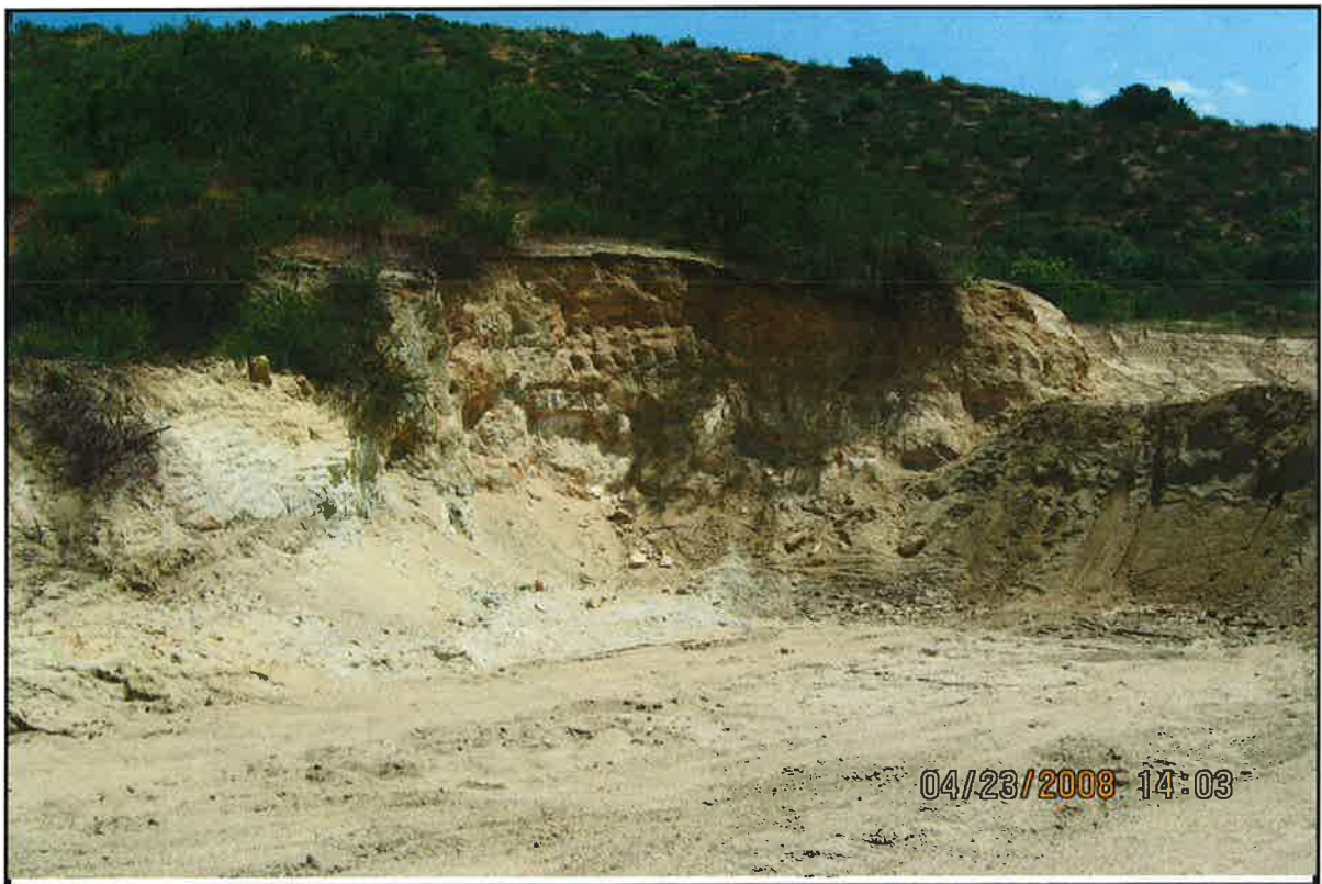
R Welch PHOTO # NOTES: Hillside excavation for track material
