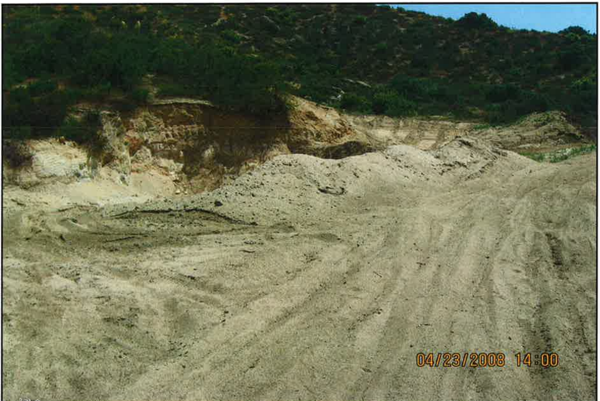
R Welch PHOTO # NOTES:4of5 showing excavation
