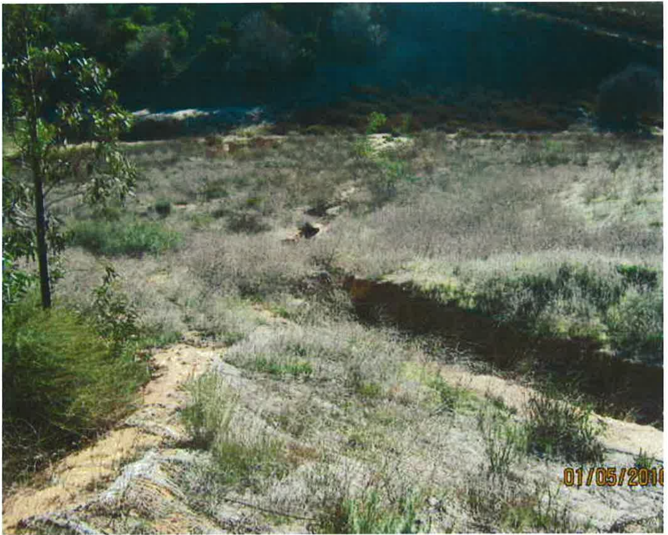
J.TATE/EROSION VISIBLE AT THE REAR OF THE PROPERTY - 01/05/2010
