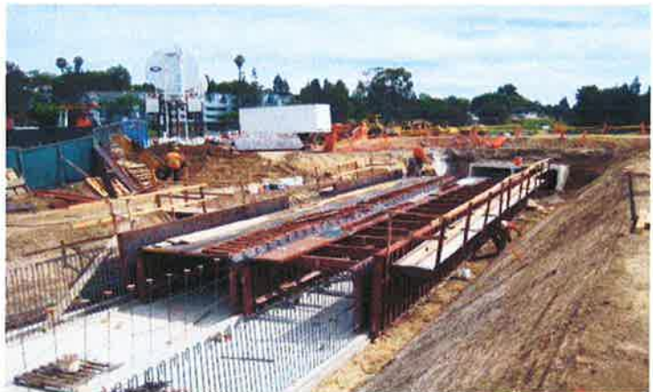
Slip form of box culvert.
