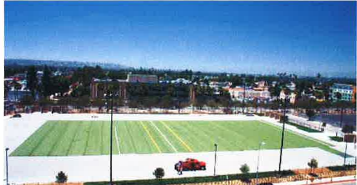
Fields during synthetic turf installation
