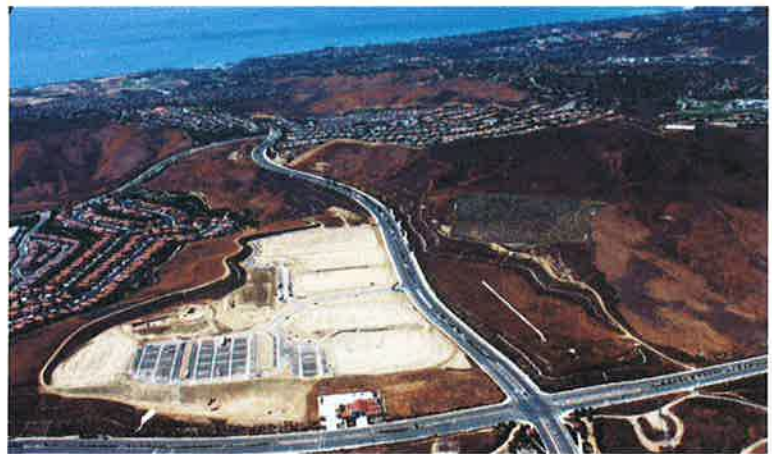
Aerial view of park in early construction
