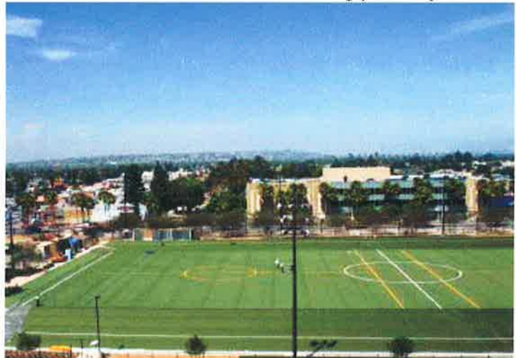
Completed installation serves as two practice or one competition field
