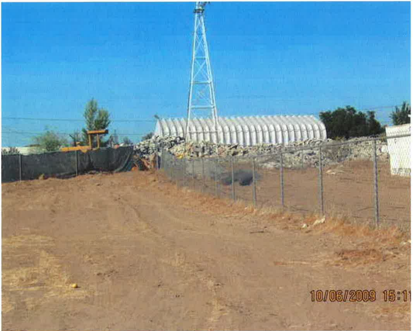
Wide shot of concrete pile looking north. J. Kirchoff - 10/06/2009
