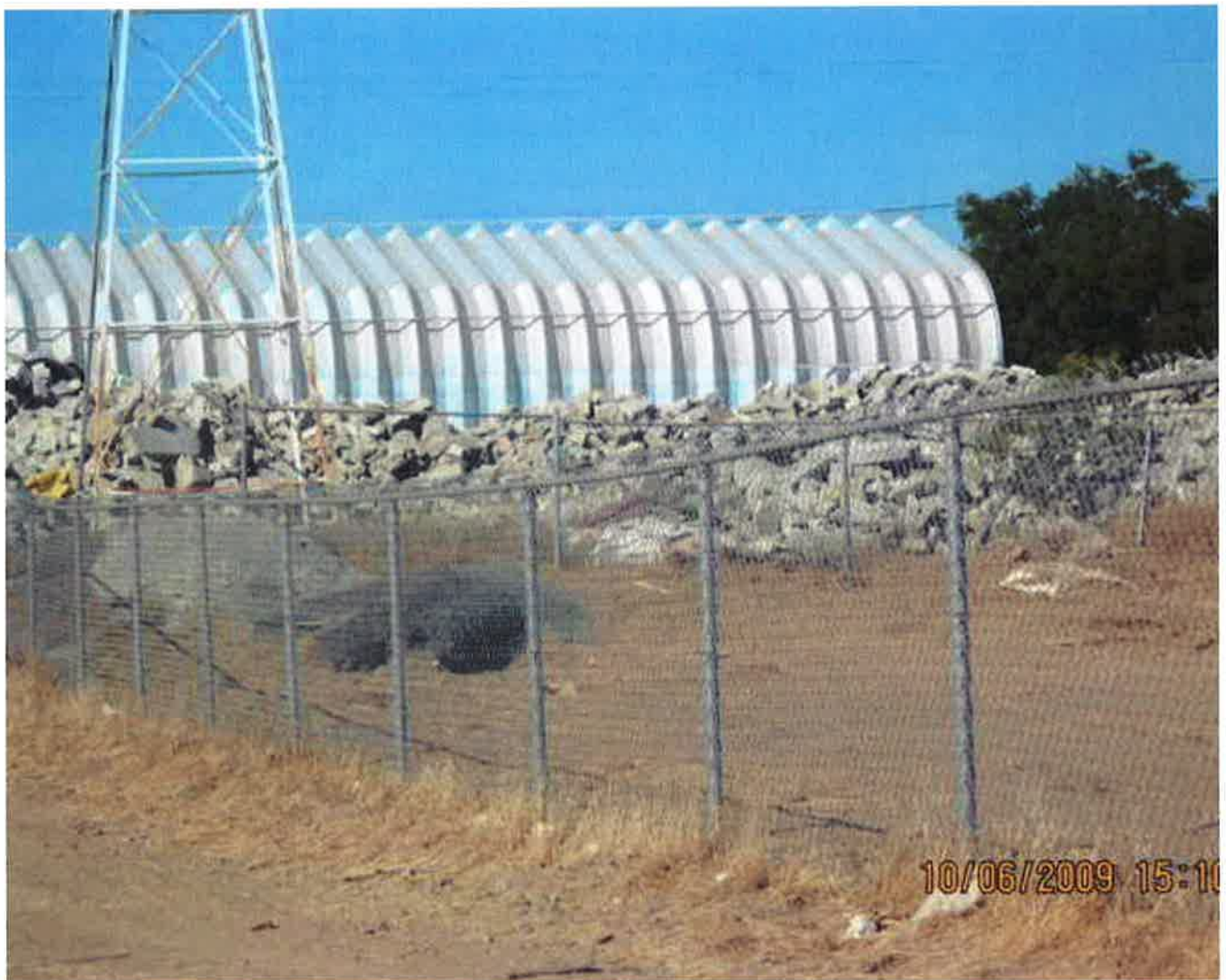
This is the first pile of broken concrete looking north. J. Kirhcoff - 10/06/2009
