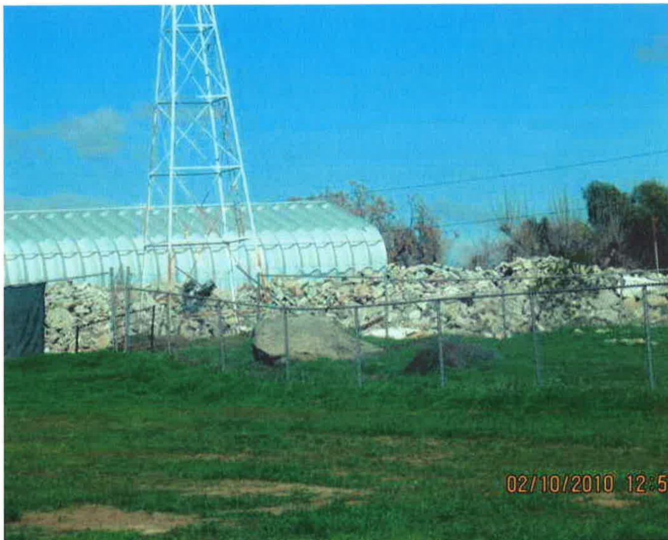
J.Wagner #80. Large pile of concrete pieces remain. - 02/09/2010
