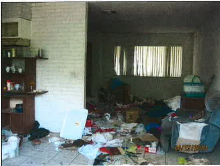
Kitchen and living area through broken window. RHannah 1100 13, 14, 17
