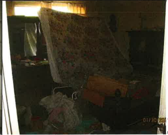
Bedroom, improper maintenance. RHannah
