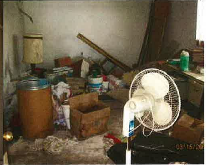
Inside of structure. RHannah NOD 14/17
