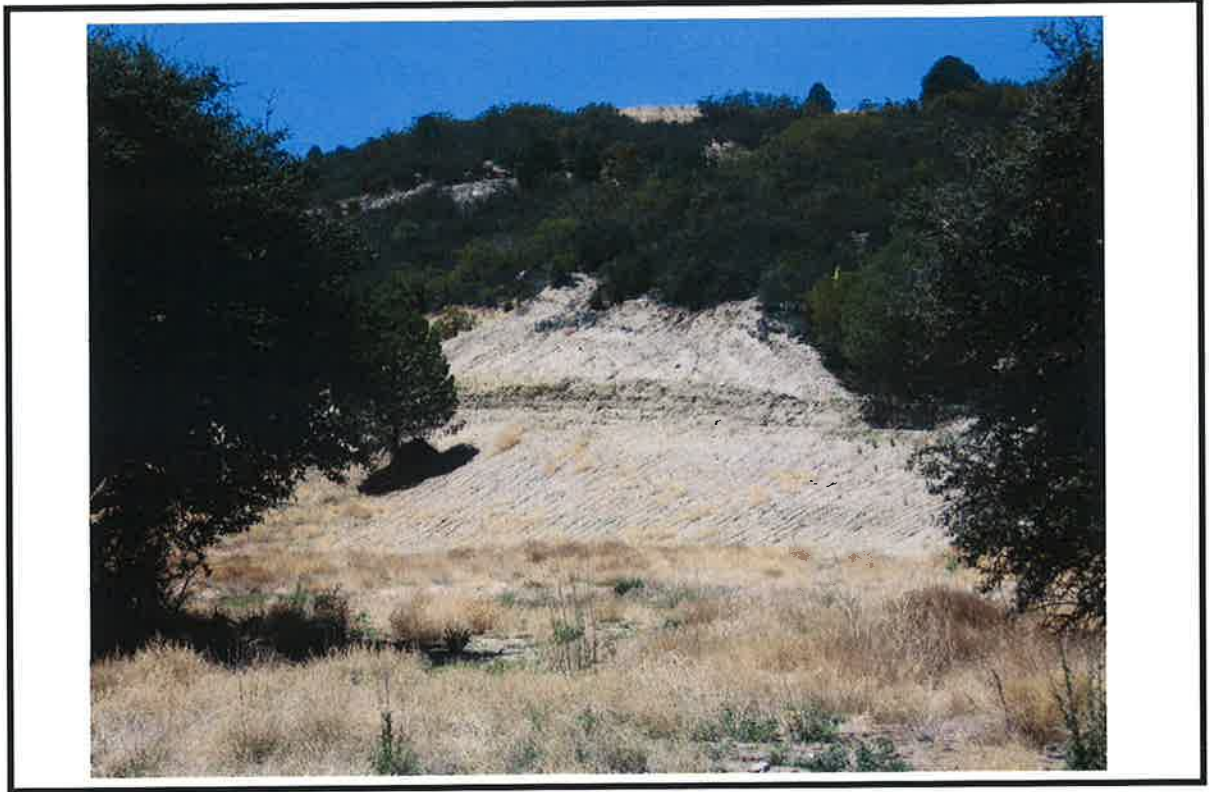
PHOTO # 1 NOTES: close up of graded road
