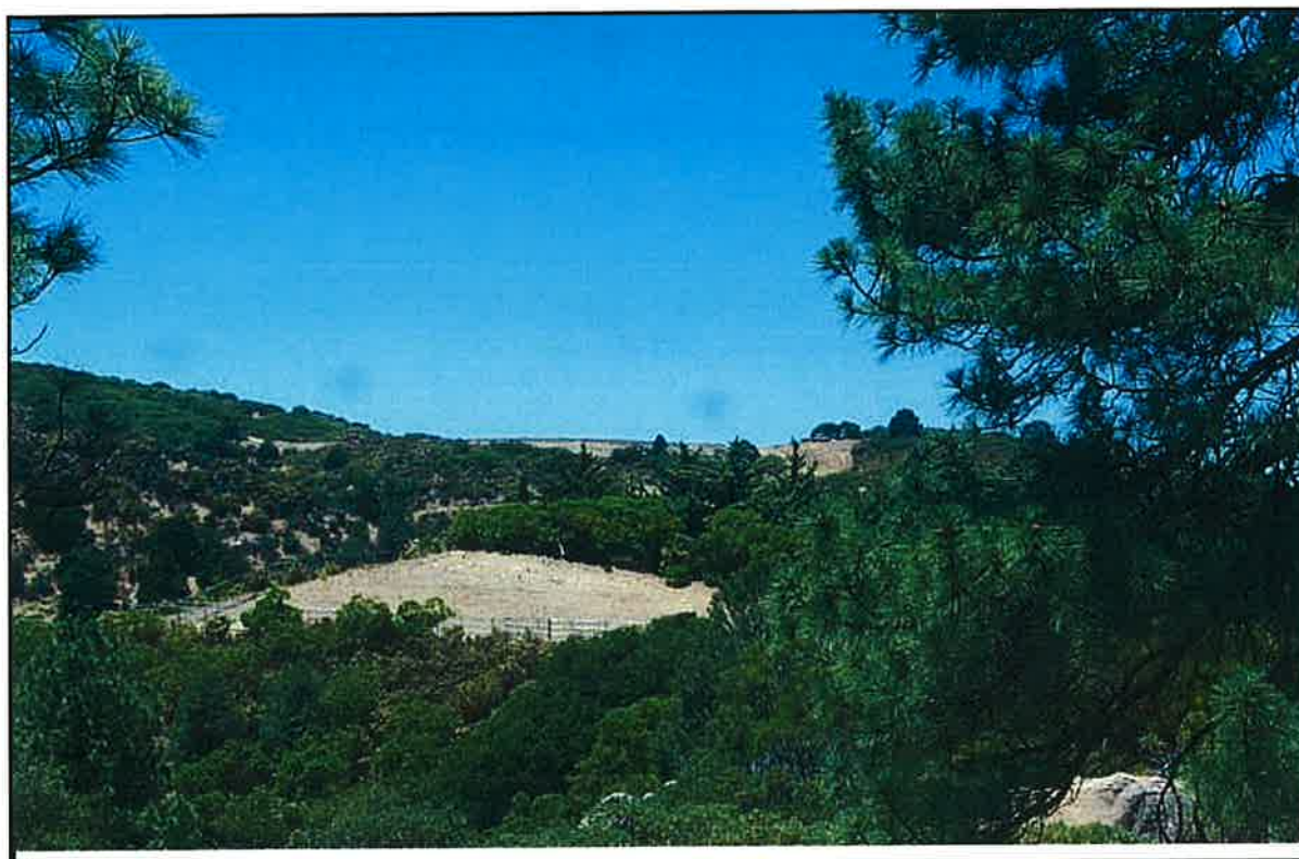
PHOTO # 2 NOTES : GRADING IN PROGRESS
