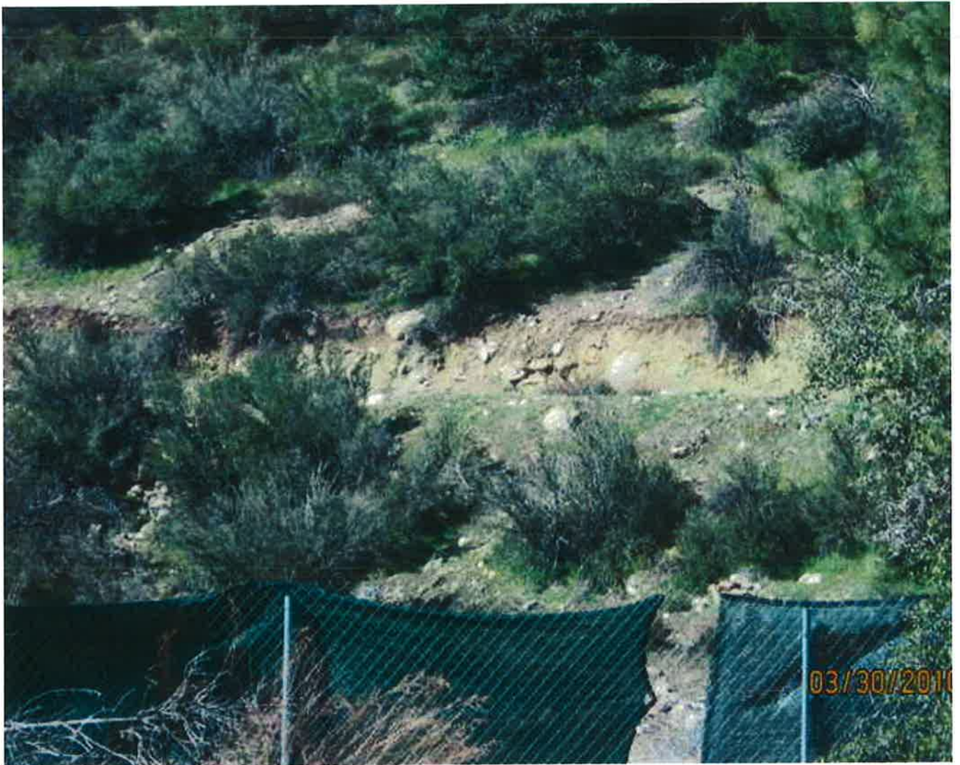
Violation remains. JHeagstedt - 03/30/2010
