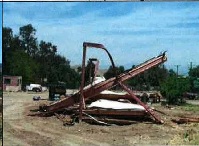
The remains of a demolished mobile unit.
