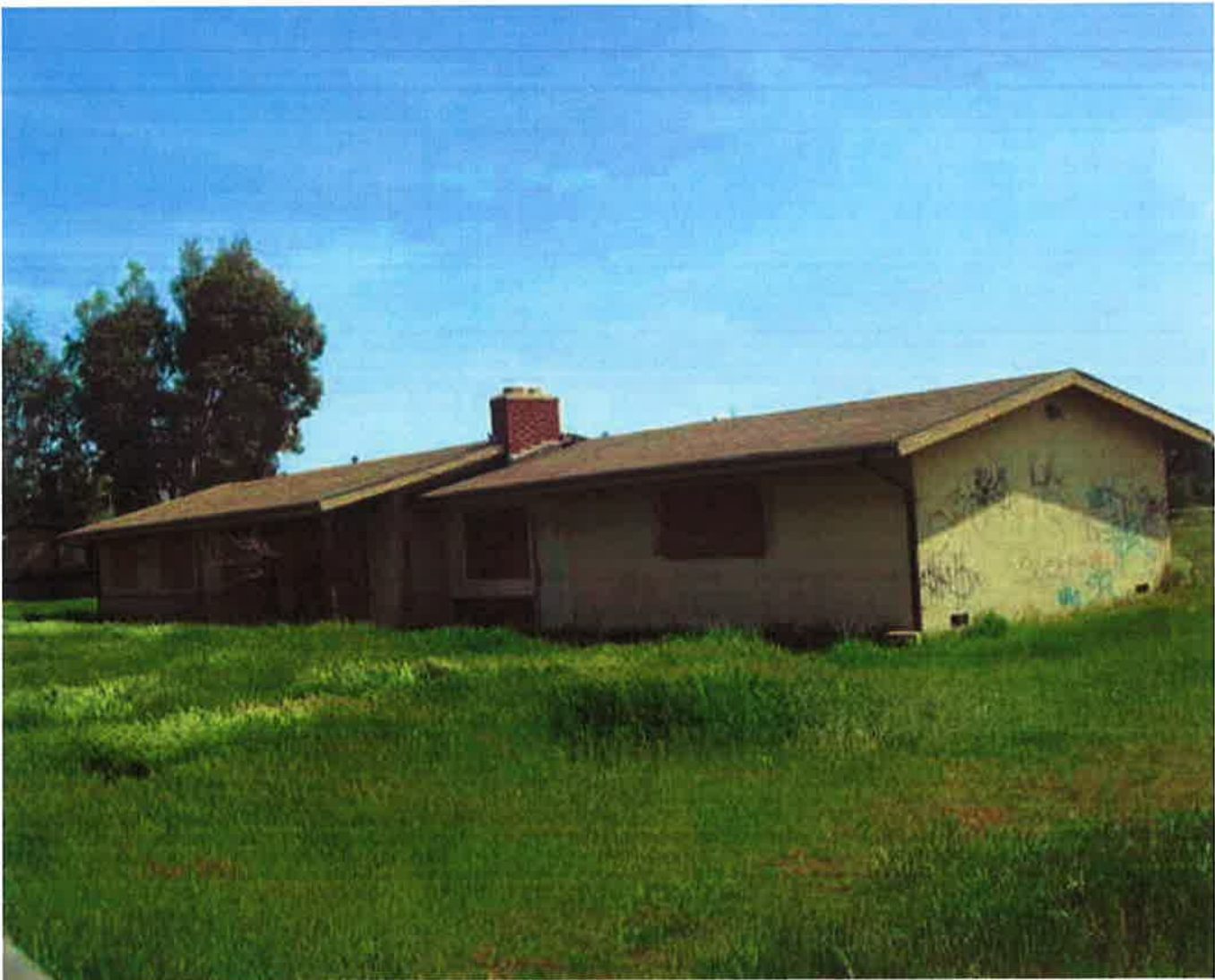
E. Torres; Structure 1 remains in substandard condition - 03/24/2010
