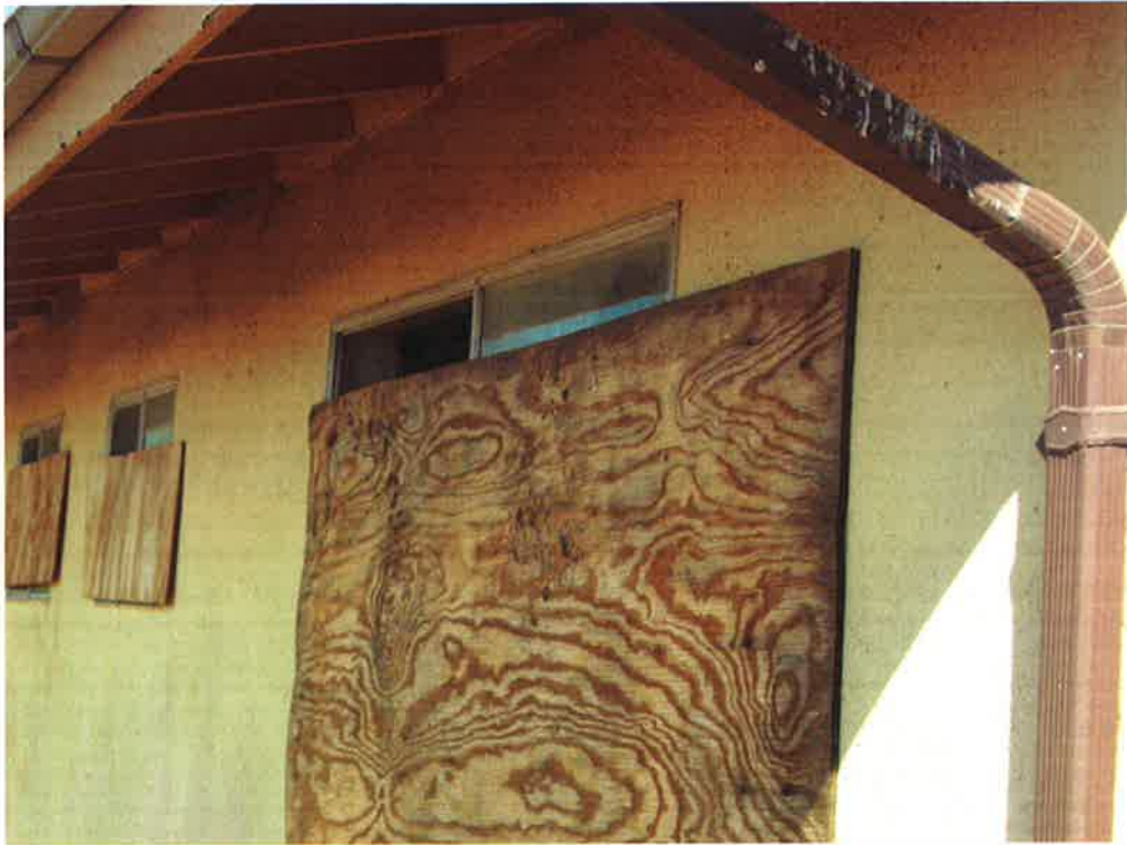
Photo 7: Structure #1 Defects 12,13,14, 17 Missing window not covered by plywood
