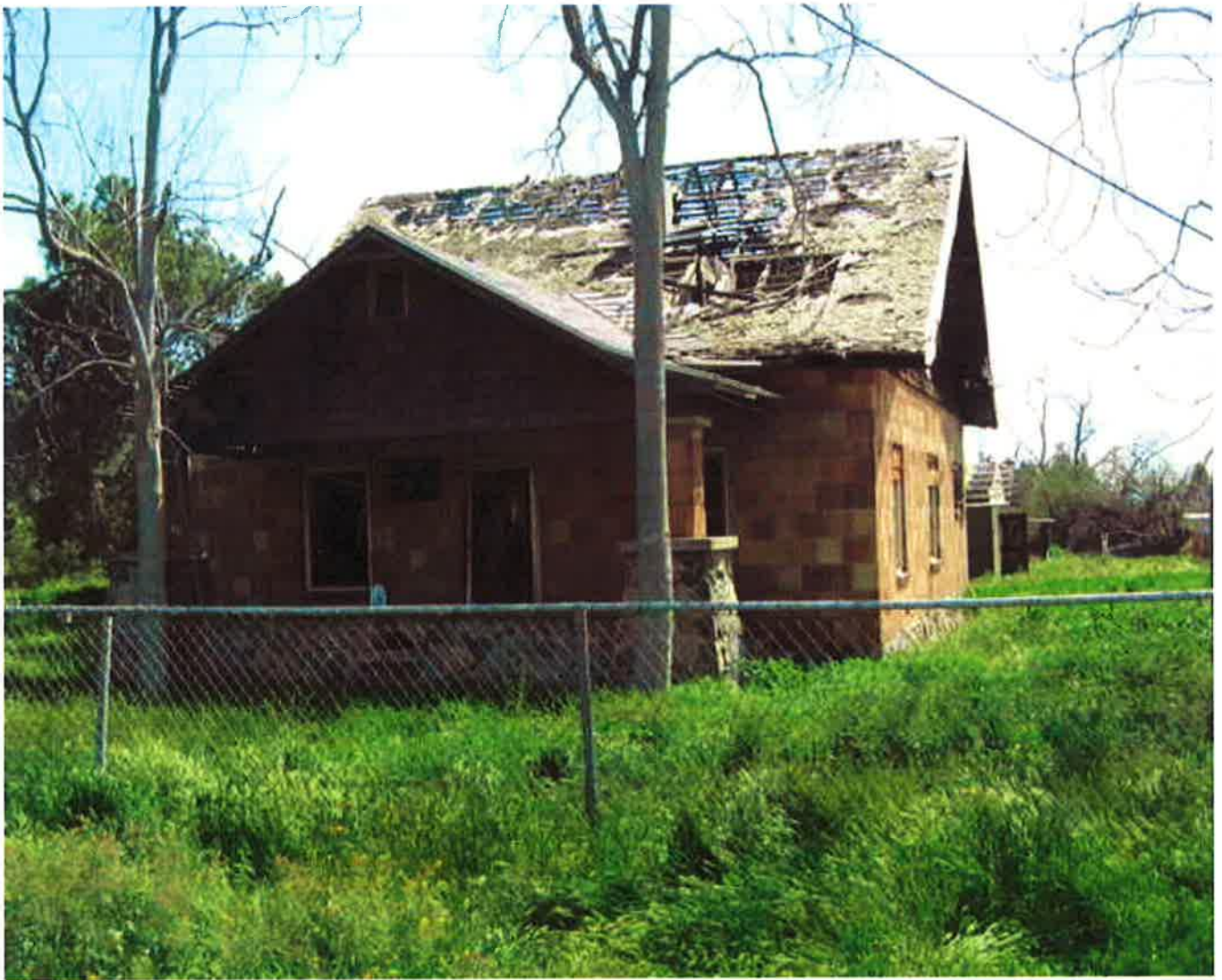
E. Torres; Structure 2 remains in substandard condition - 03/24/2010
