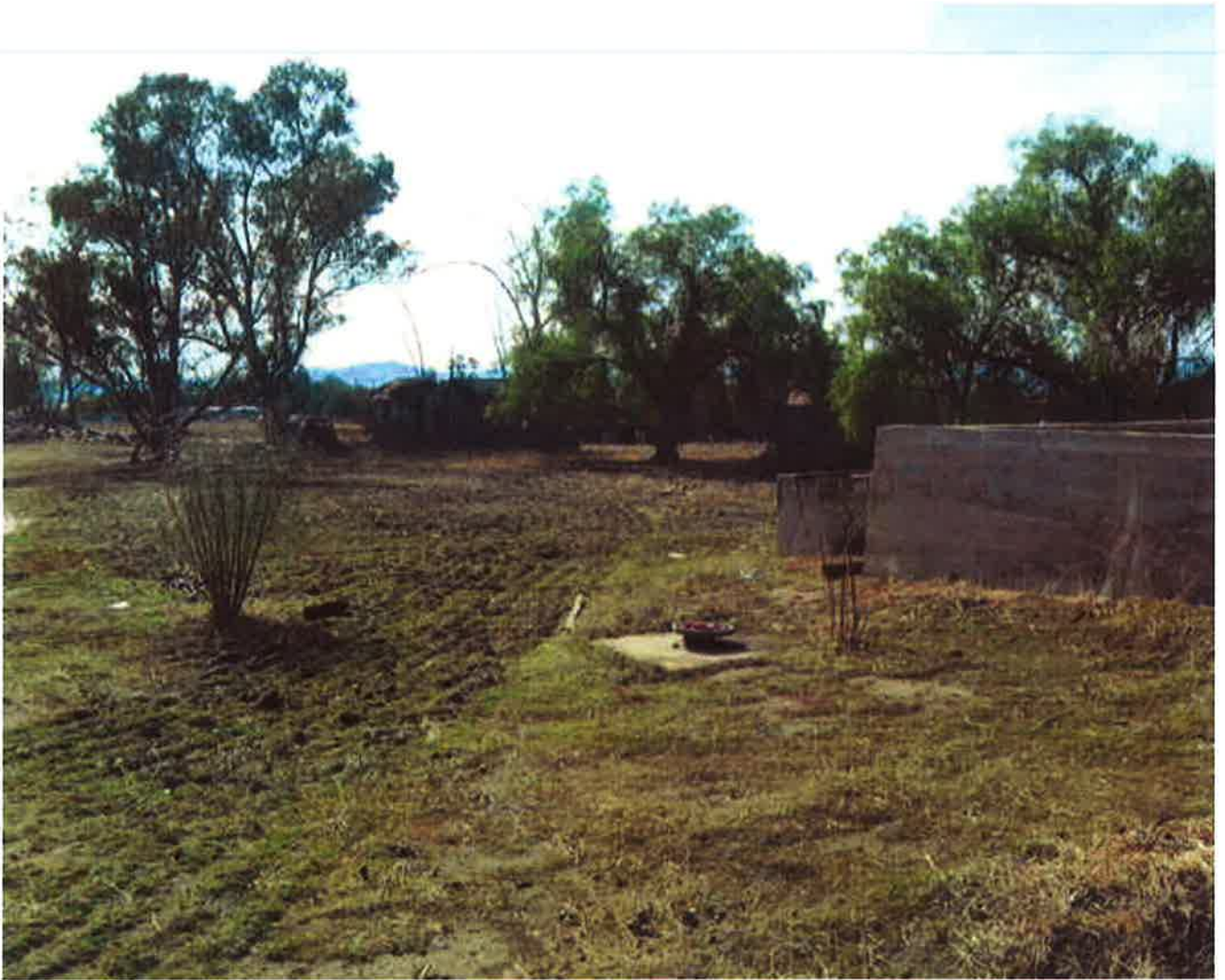
E. Torres; Structures 4 & 5- no change - 12/16/2009
