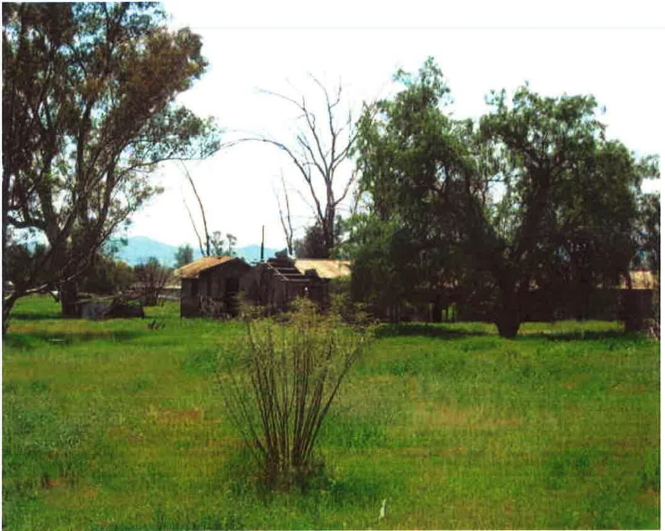
E. Torres; Structures 4 & 5 remains in substandard condition - 03/24/2010
