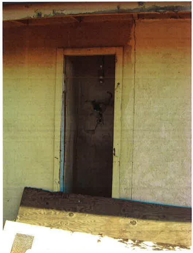
Photo 7: Structure #1 Defects 12,13,14, 17 Missing window not covered by plywood
