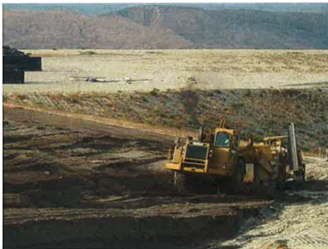
GeoSyntec performed construction quality assurance services for Phase 2A Module 1 construction.
