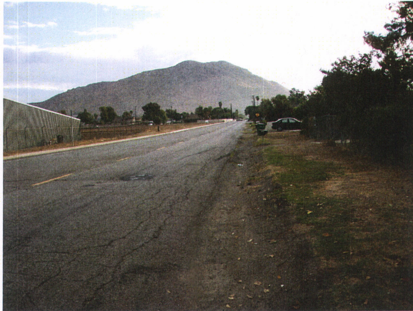
Photo 3 - View of Main Street eastward towards Michigan Avenue.
