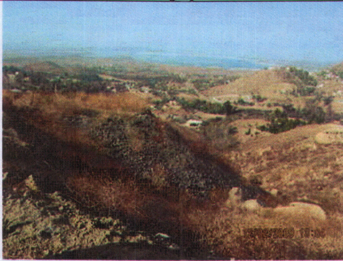
Grading on hillside
