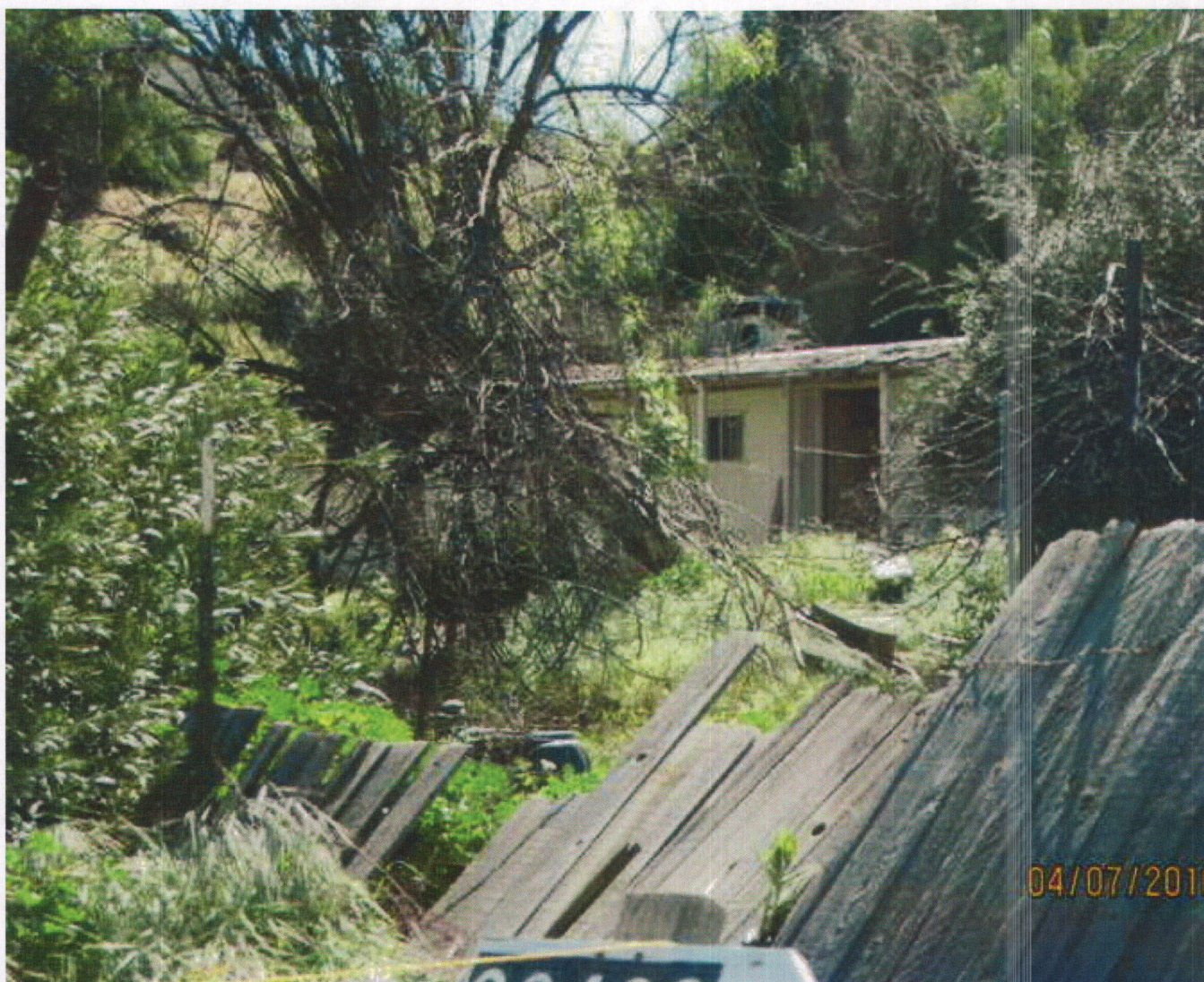
R Ryder - the violations of AR / EOS remains on the property - 04/07/2010
