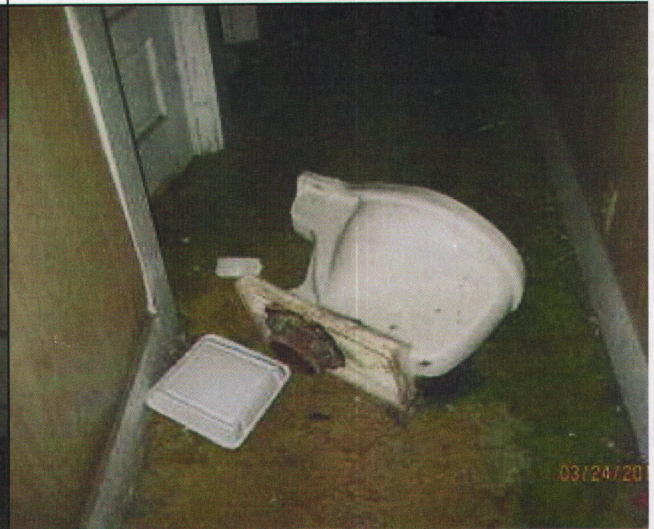
M Sanders 024510 SSS # 1 - toilet pulled from bathroom
