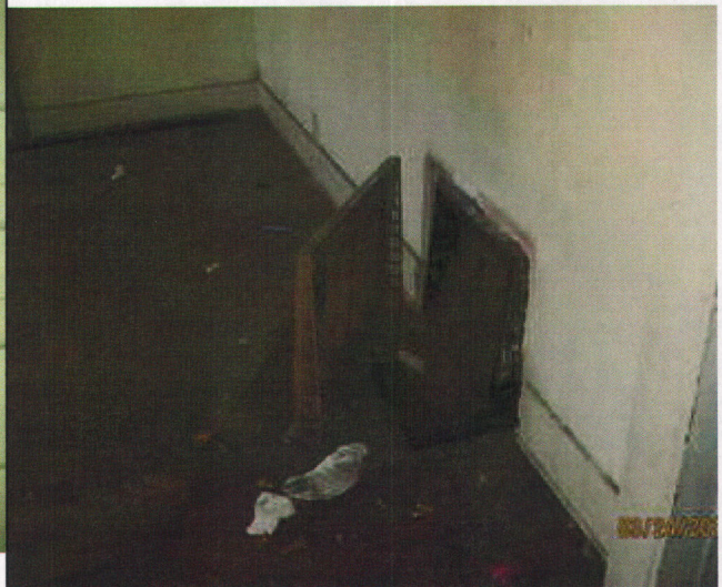
M Sanders 024510 SSS # 1 - dismantled floor he
