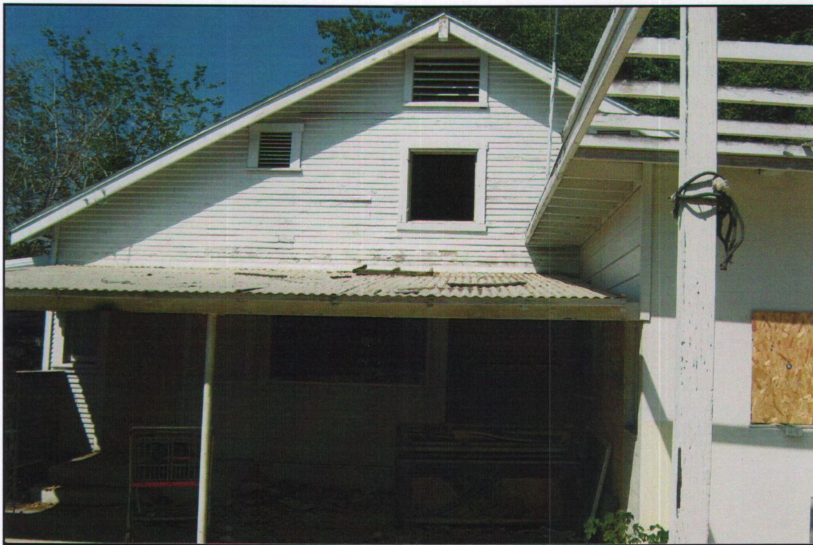
PHOTO #5 Rear of dwelling w/open upper window.
