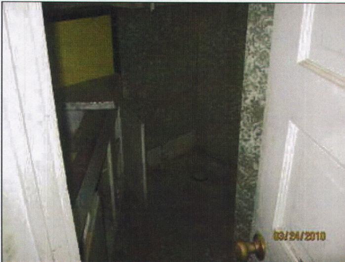
M Sanders 024510 SSS # 1 - missing toilet
