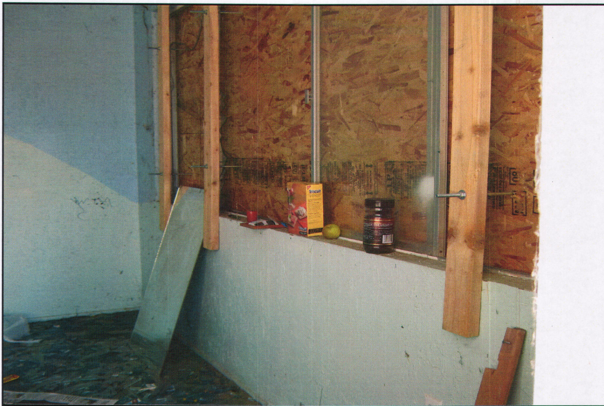
PHOTO #3 Interior of room where sliding glass window shows habitation.
