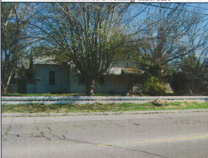
Distressed dwelling unit. KR
