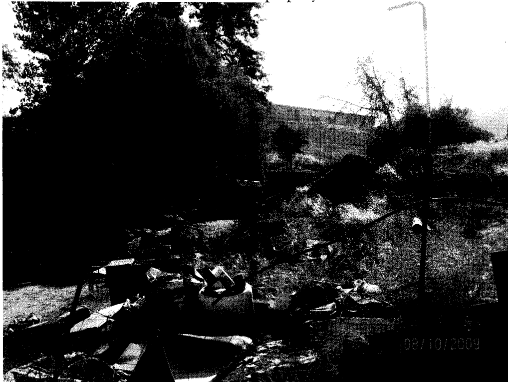
PHOTO # 2 NOTES: Violations remain on the property
