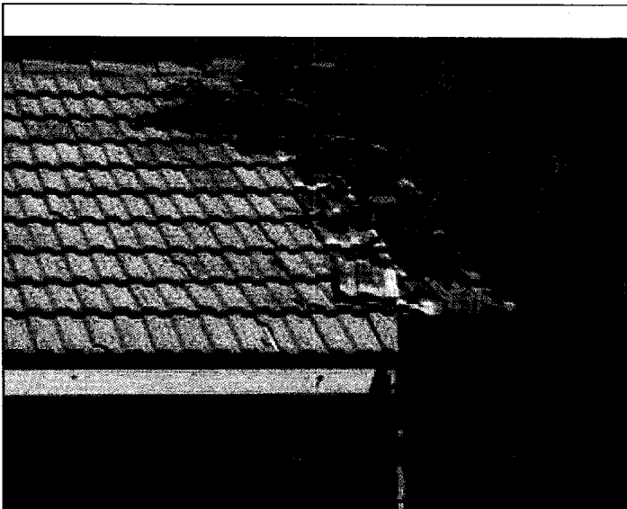
M Sanders 040610 - missing roof tiles SSS #2
