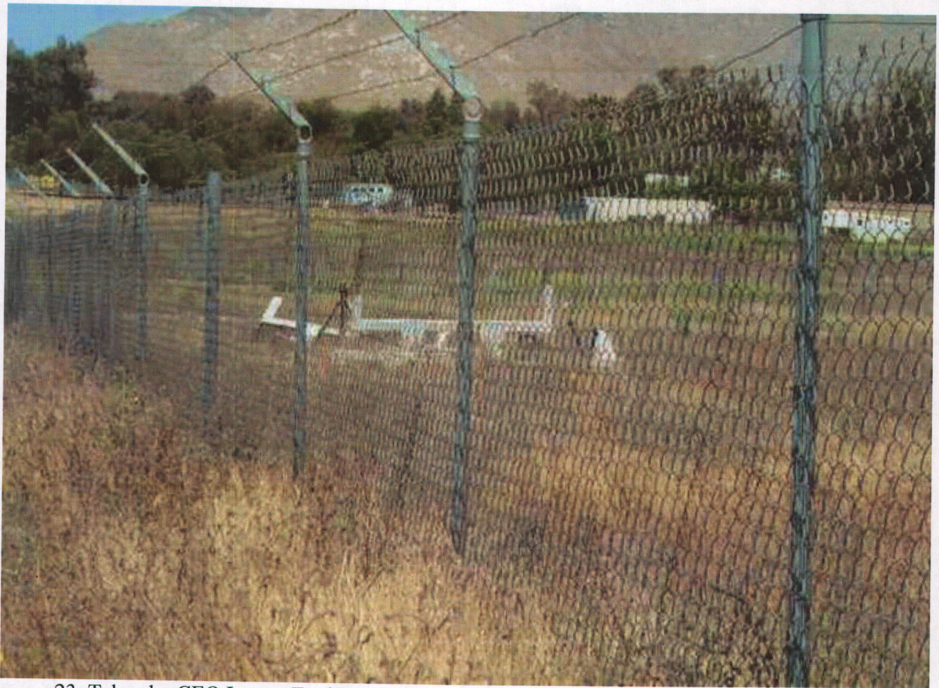
23. Taken by CEO Lyon - Equipment parts remain along the south side of the property. - 05/04/20
