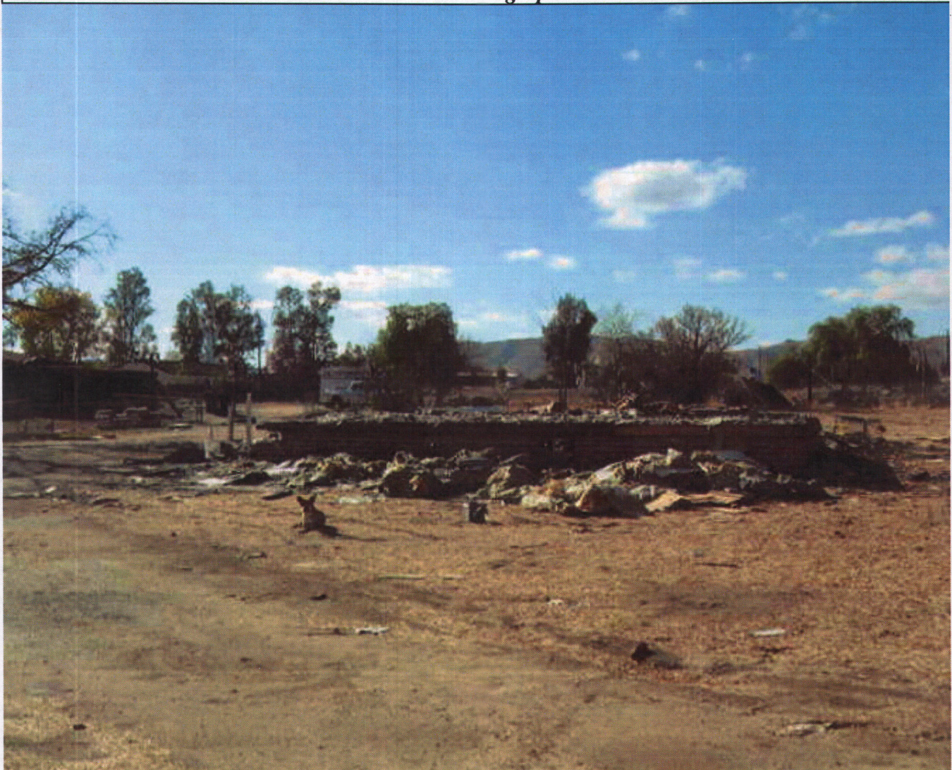
CV09-05589 Substandard structure - photo #1 - 12/08/2009
