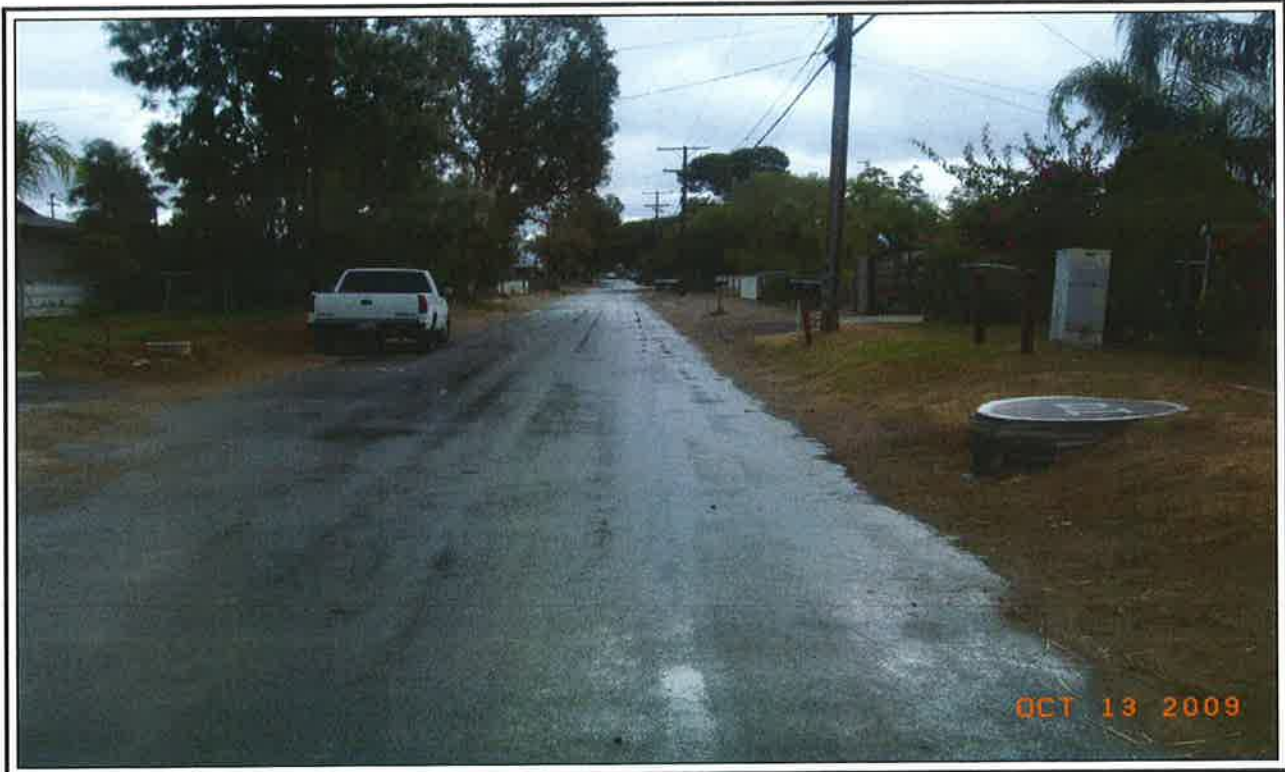
Figure 5. Day Creek - Frank Ave Storm Drain: Frank Avenue looking south (just north of 65th Street)
