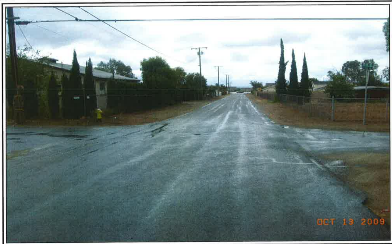
Figure 6. Day Creek – Frank Avenue Storm Drain: Intersection of 65th Street and Frank Avenue (65th Street looking west)
