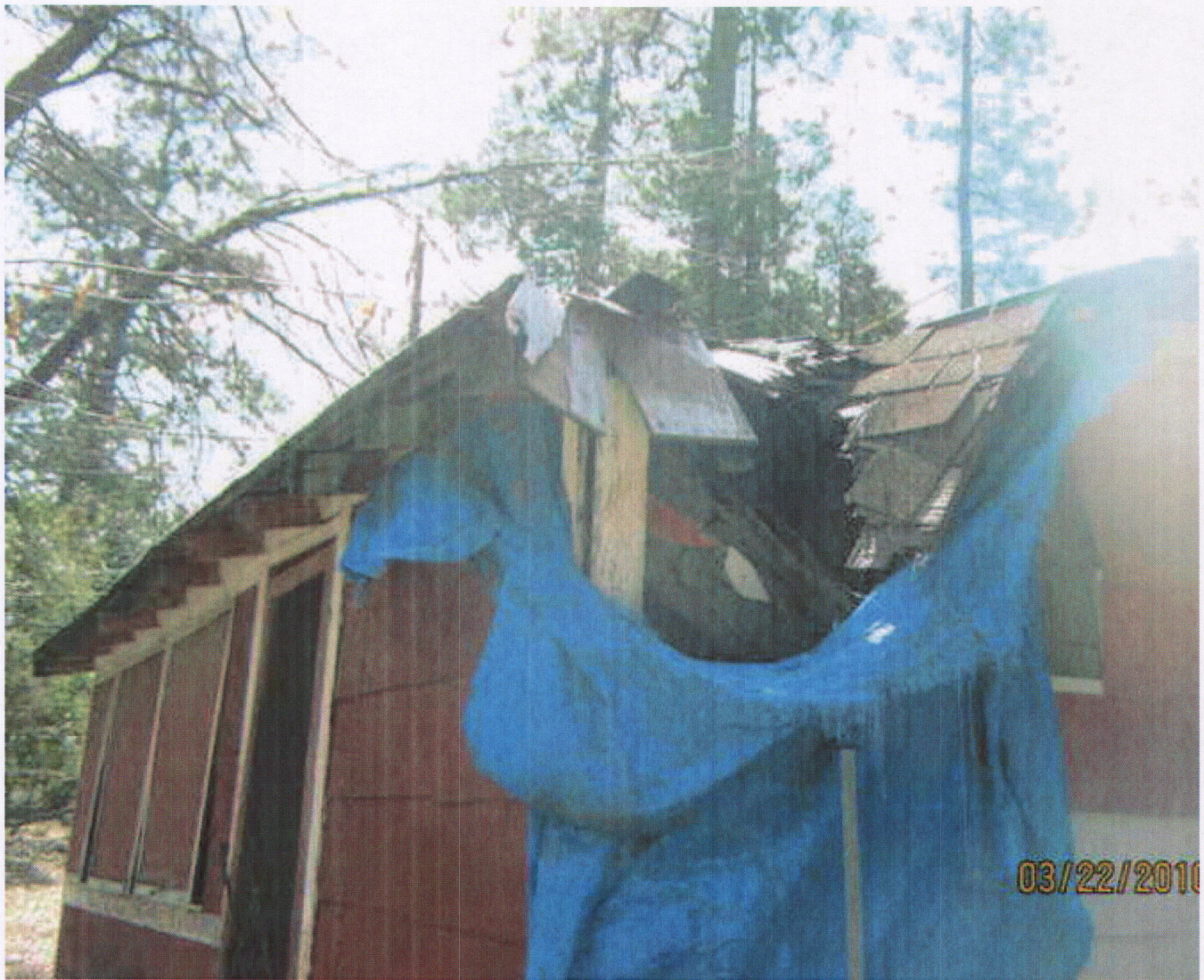
CForrey / Defect #10, 11, 12 Open, damaged roof and walls - 03/22/2010
