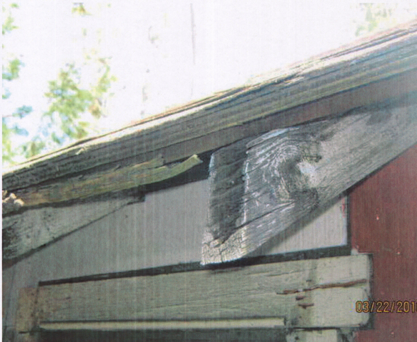
CForrey / Defect #14, no mainenance, eaves deteriorated - 03/22/2010
