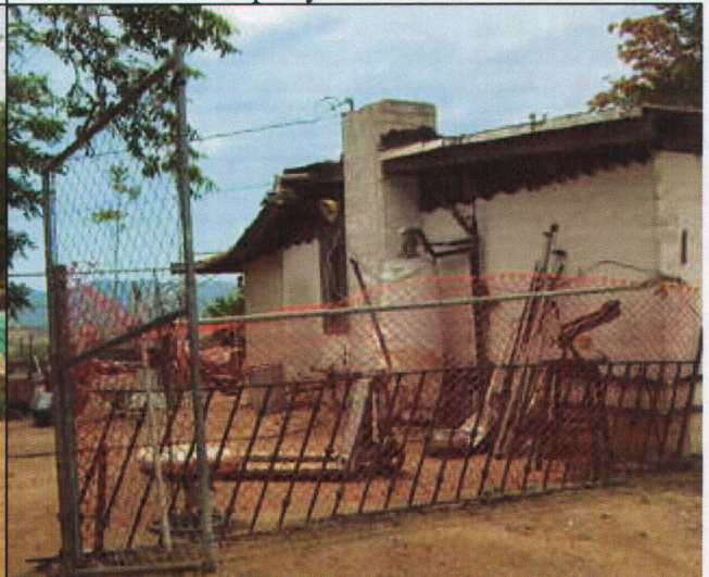
05/13/10 - Property Remains in Violation – Pike
