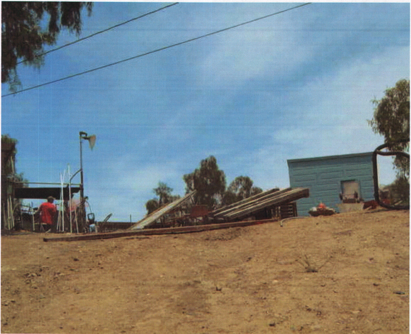
05/13/10 - Property Remains in Violation - Pike - 05/13/2010
