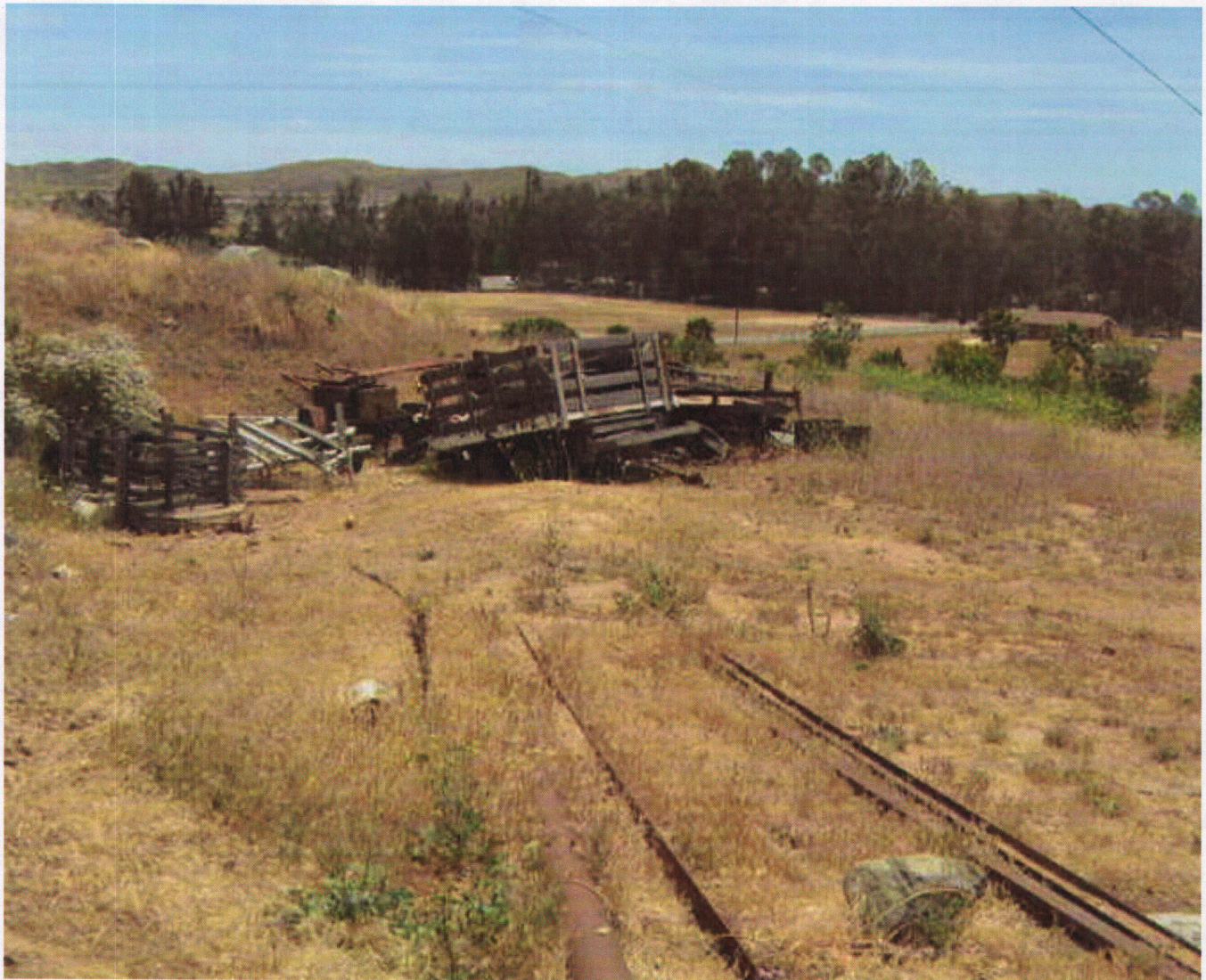
05/13/10 - Property Remains in Violation - Pike - 05/13/2010
