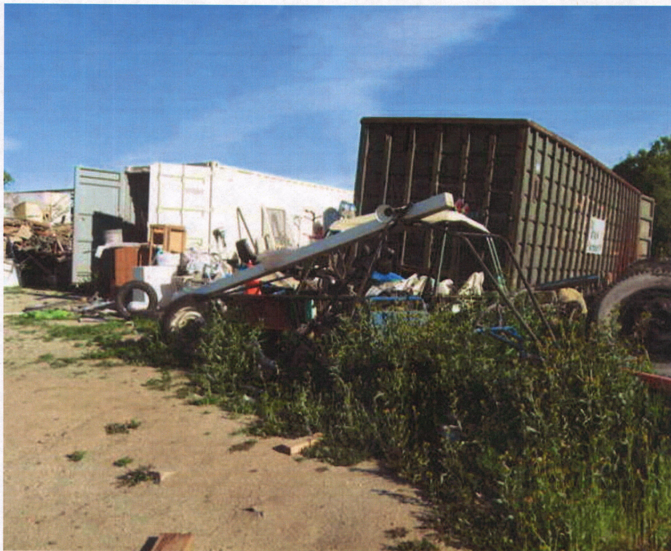
Rubbish, shipping container and Outside storage remain-JMorris - 03/16/2010
