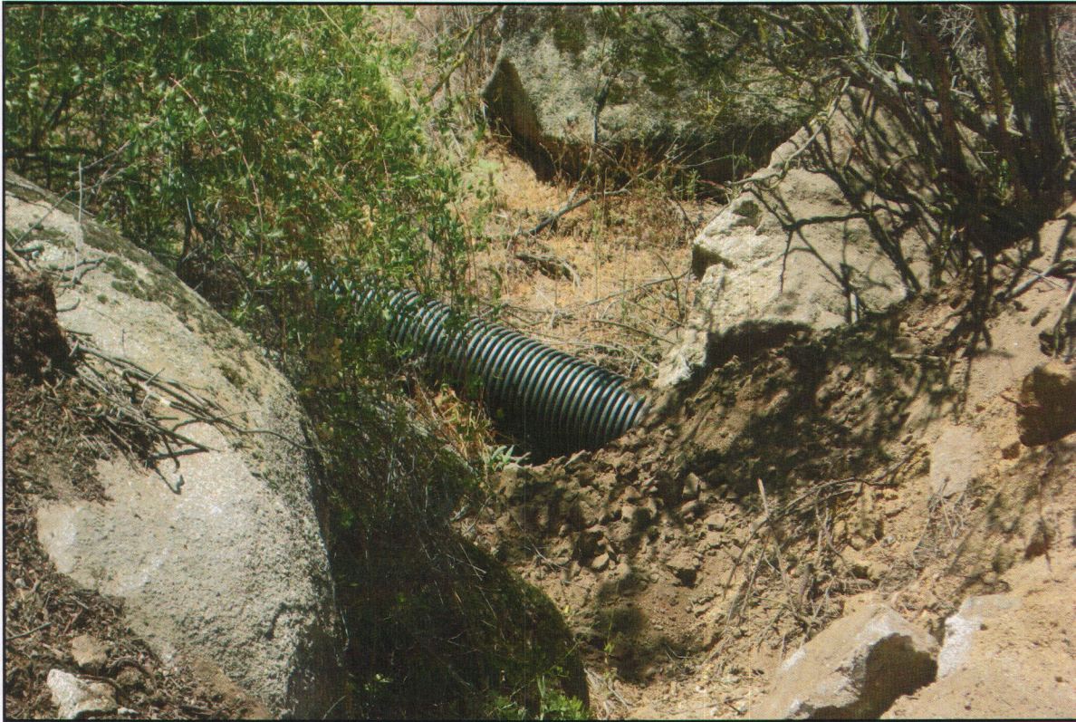
PHOTO #3 Culvert piping placed through the rock. 05/13/08
