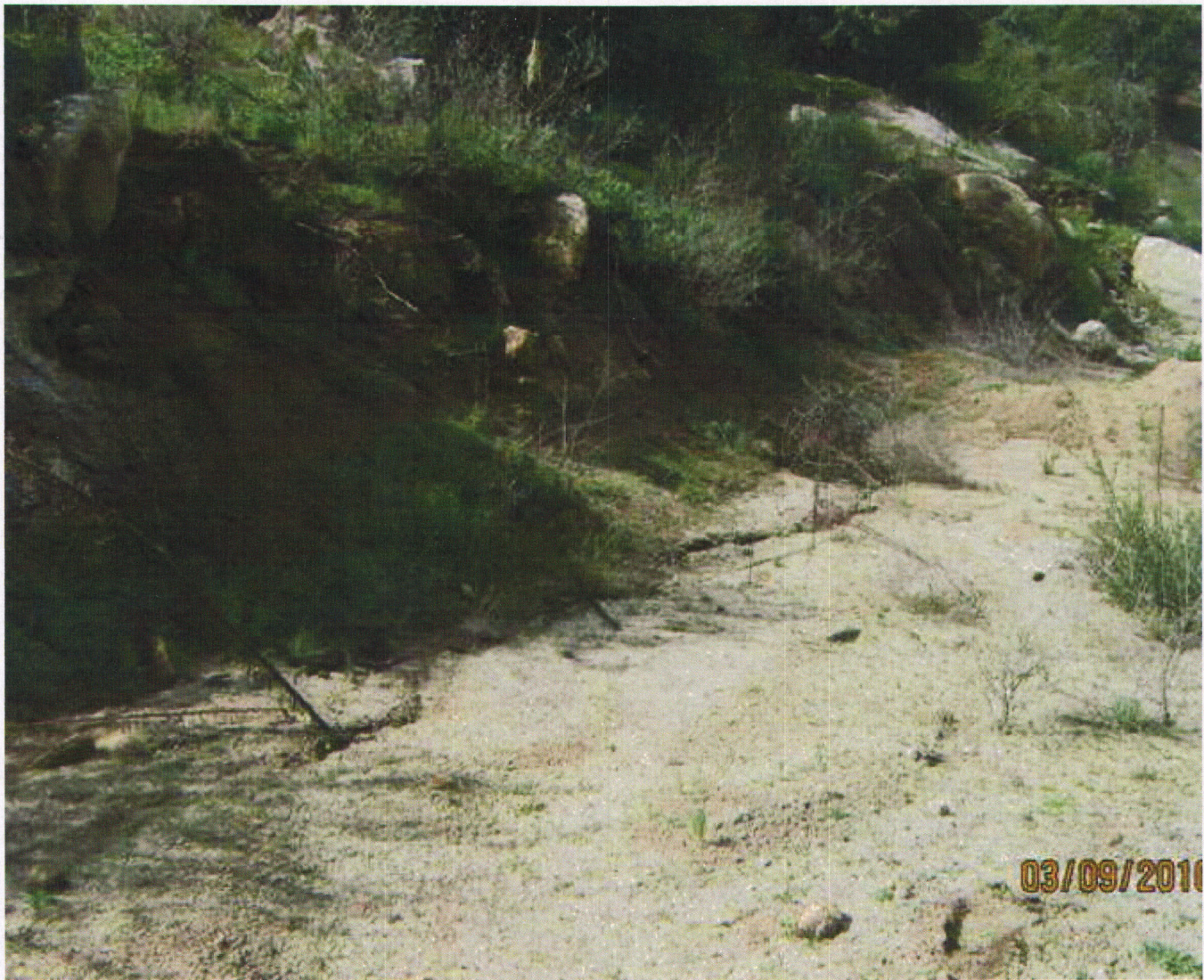
B POLLARD 030910 cwp-CUT INTO HILLSIDE - 03/09/2010
