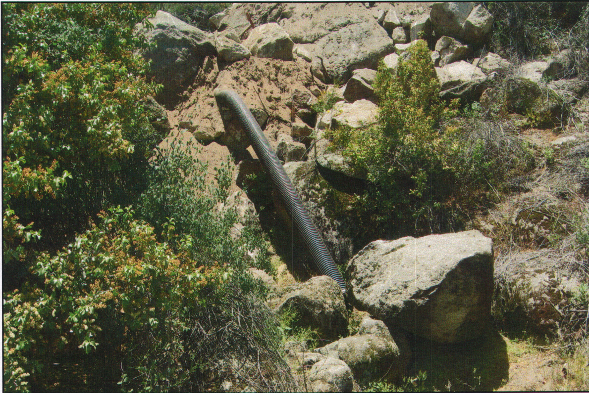
PHOTO #9 Culvert coming through rocks. 05/13/08
