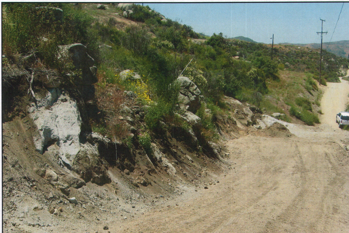
PHOTO #6 Hillside cut into from grading process on alternate road.
