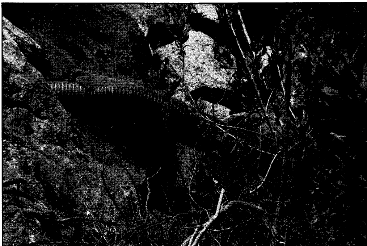
PHOTO #2 Culvert piping placed through the rock.
