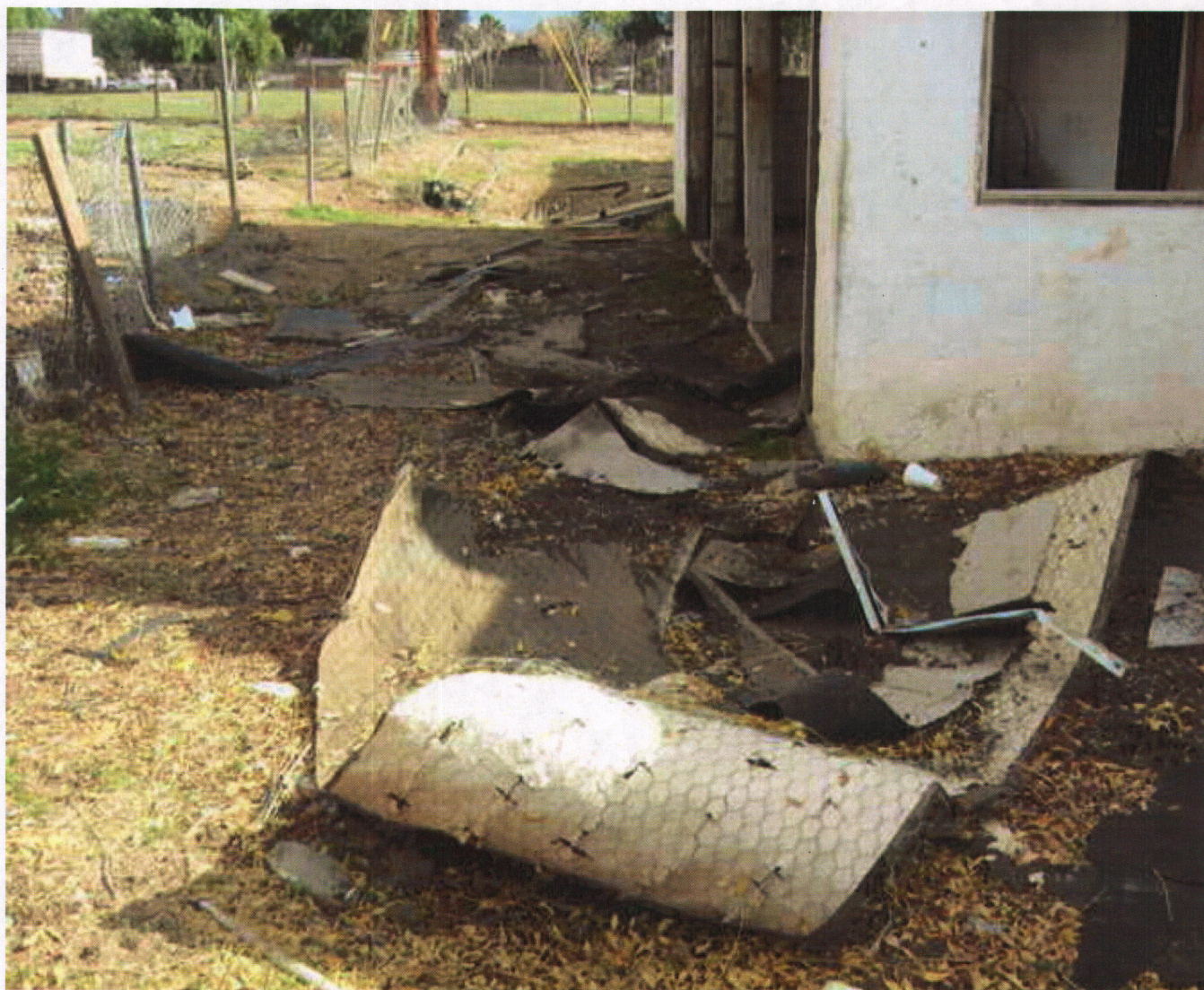
Rubbish remains on the property-JMorris - 01/12/2010
