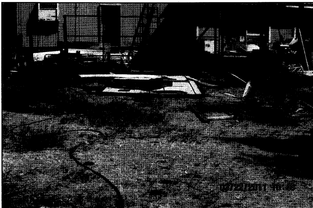
Photo # 10 Date: 03/22/11 Time: 10:40 AM Taken By: T Cervantes 6
