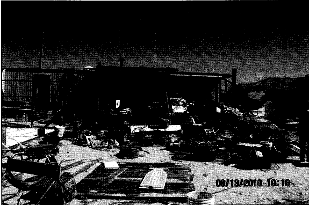
Photo # 3 Date: 08/13/10 Time: 10:18 AM Taken By: T Cervantes
