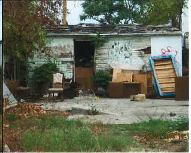
W. Jose - Back of Structure
