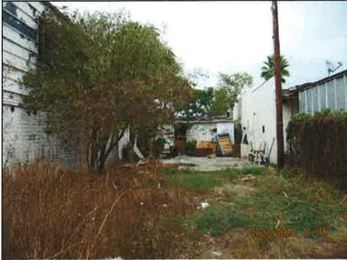
W. Jose - Back of Structure
