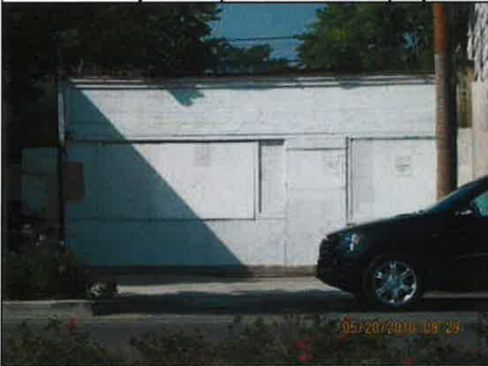
N. Wapner - Front of Property
