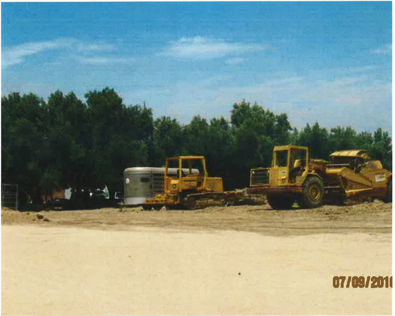
J Chamberlain/Follow up, grading equipment present - 07/09/2010
