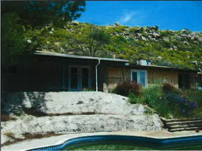
Vacant, abandoned main dwelling unit. KR
