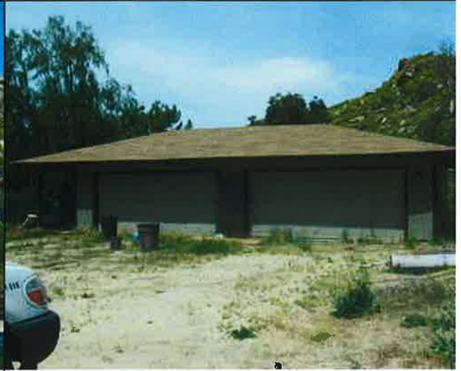
Vacant, abandoned 4 car garage. KR
