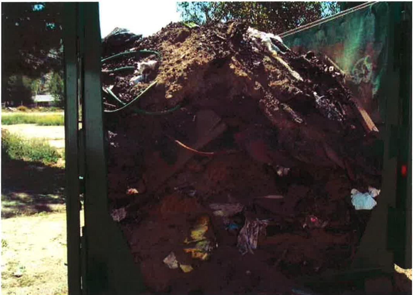
Taken by CEO Lyon - The owner was suppose to off load the concrete and dirt from this dumpster so it c dumped but they have not even attempted to do it. - 04/19/2010
