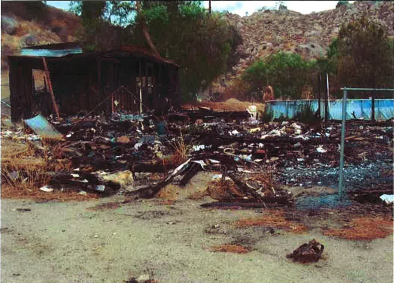
Taken by CEO Lyon - The mobile that was on the property is completely burnt and the debris is through fenced in front yard. - 11/13/2009
